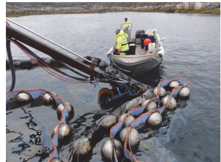
Collecting burning residue with Bucket Skimmer, Greenland
