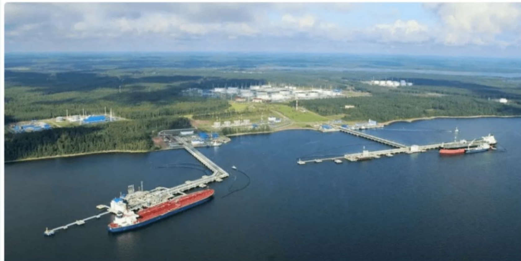
Primorsk Oil Terminal, image credit:unn.ua
