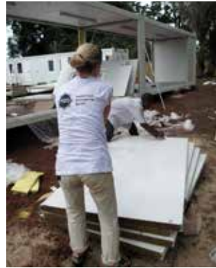
The erection of a fully equipped prefabricated camp in northern DRC.
