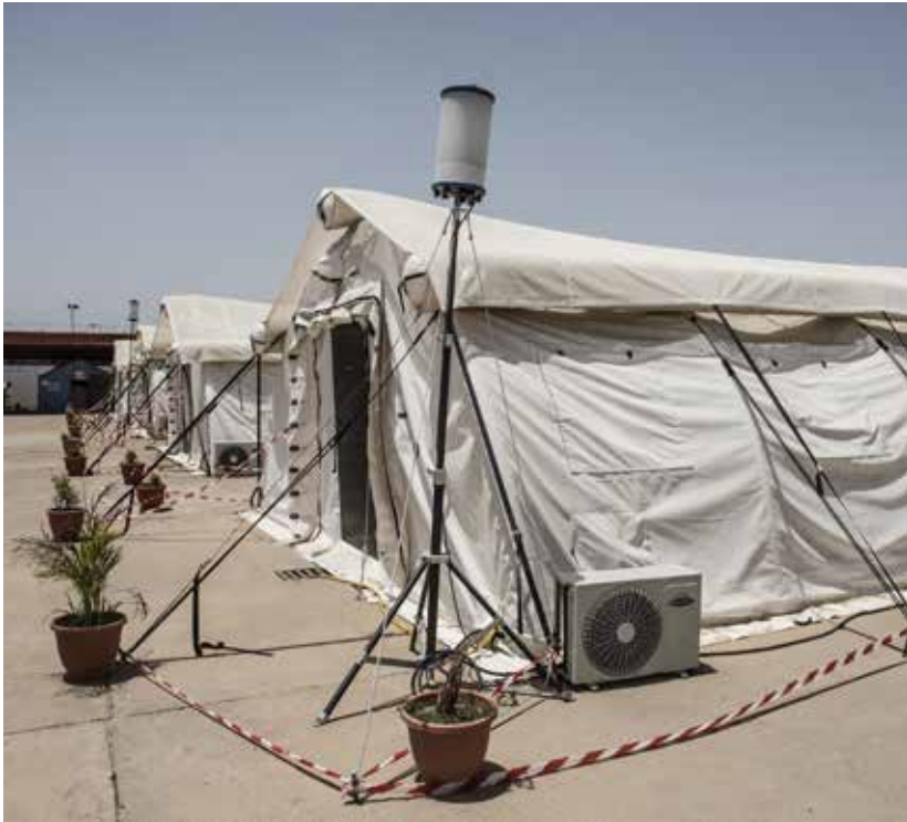
MSB/IHP base camp Red Roof in Maiduguri, Nigeria. The camp consists of safe accommodation, offices, sanitary facilities, kitchen, water purification, electricity and power distribution, medical facilities etc.
