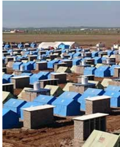
MSB shelter support in Dohuk, Iraq.
