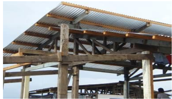
Roof construction vulnerable to wind
