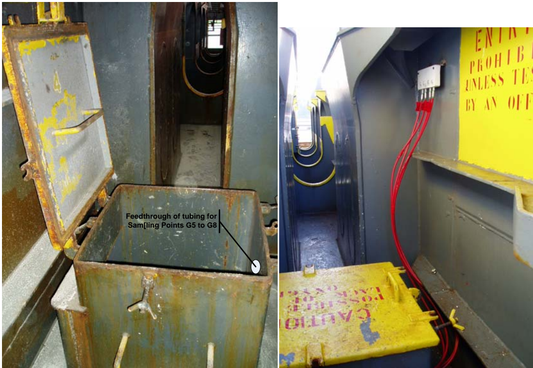
Picture 3.3.3 Stairway access hatch opening
