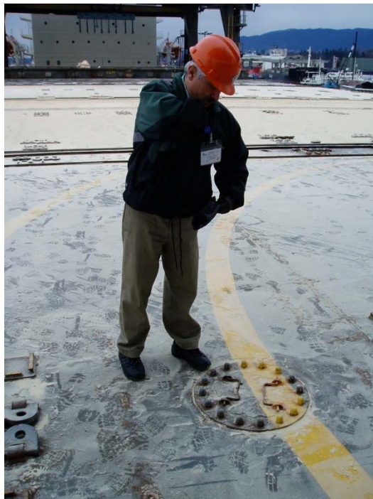
Picture 3.4.2 Cement hole cover in pontoon and mounting of Rh_2
