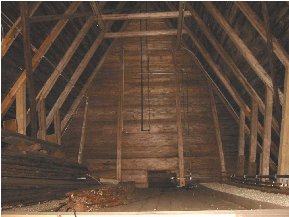
The attic of the church. Photo: Anders Lönnermark.
