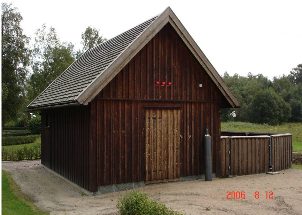
The new built building outside the church yard that contains the gas driven pump (GPU) and the water reservoir.
