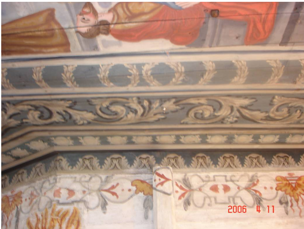
One of the high-pressure water mist nozzles at the ceiling, seen from a distance.
