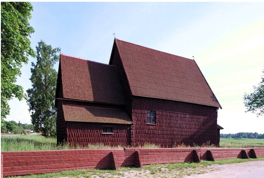
Figure 1 The Södra Råda church was completely destroyed in a fire in November 2001. Photo: Swedish National Heritage Board.
