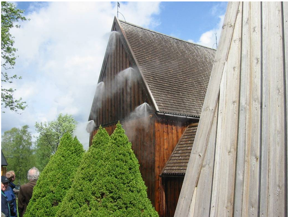
Functional test of one of the sections that protects the facades of the church. Photo: Anders Lönnermark.
