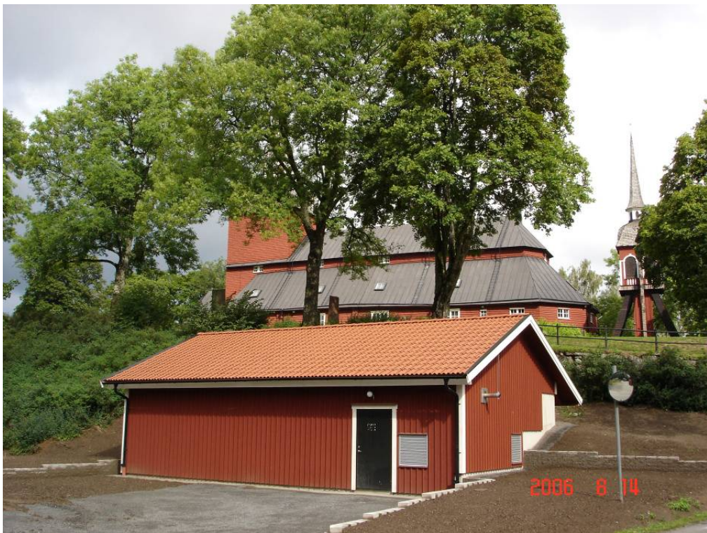
The newly built building close to the church that contains the pump units, the diesel generator and the fresh water tank. The building is insulated and heated.
