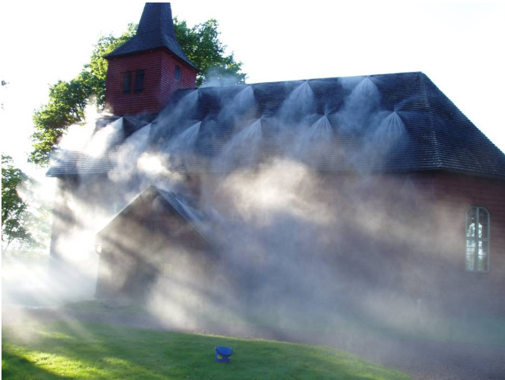
Figure 10 Protection of the facades and the roof of Älgårds church using a water mist system. Photo: Jan G Andersson.
