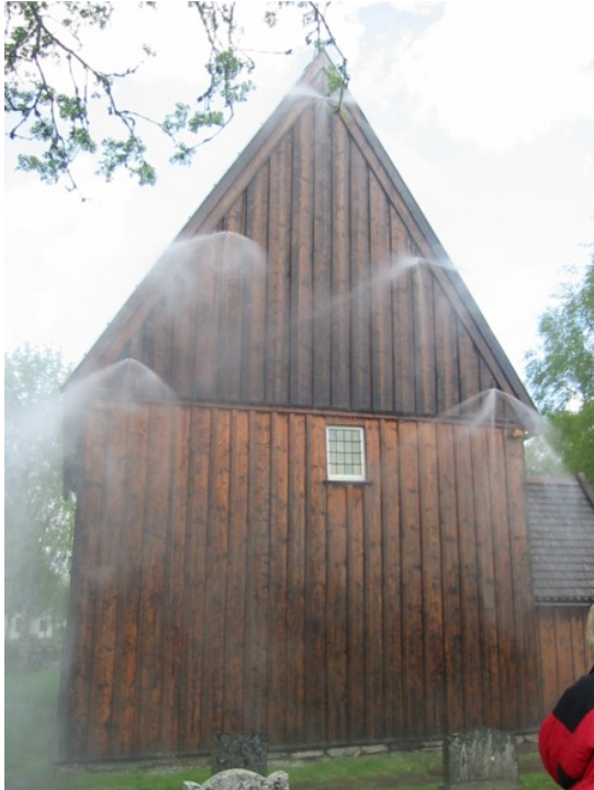
Functional test of one of the sections that protects the facades of the church. Wind velocity was high during the test; however, the water spray from the nozzles was not significantly affected. Note: The water spray provided a more uniform and higher degree of wall wetting than indicated by the photo. Photo: Anders Lönnermark.
