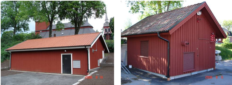
Figure 4 Buildings built close to the churches that contain the water reservoir, pumps and associated equipment. To the left is the building for Habo church and to the right the building for Älgårås church.
