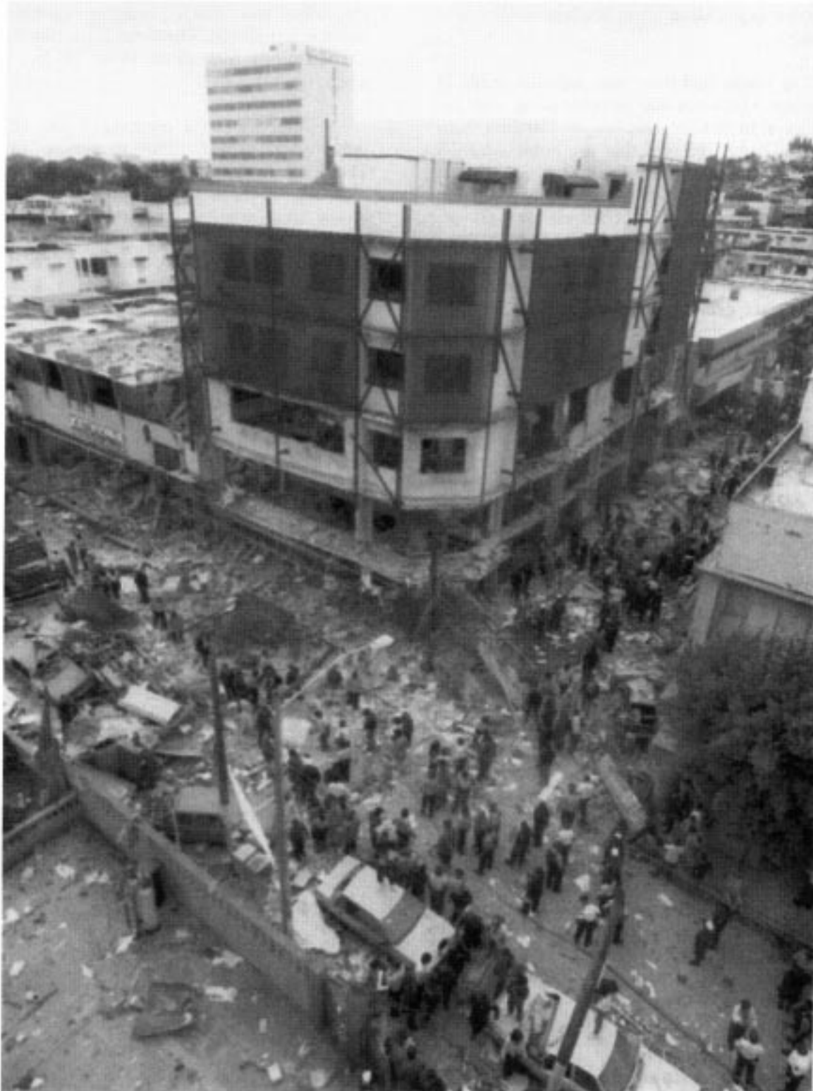
Figure 3. Building after Explosion (courtesy of The San Juan Star ).
