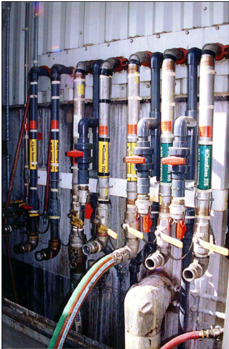
Figure 2. Transfer coupler access panel with transfer hose attached
