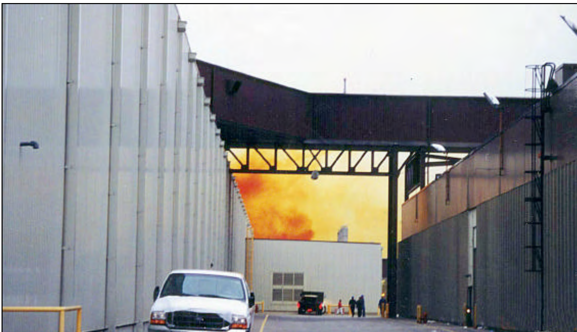
Figure 1. Postaccident view of the bulk storage building (center) with vapor cloud visible
