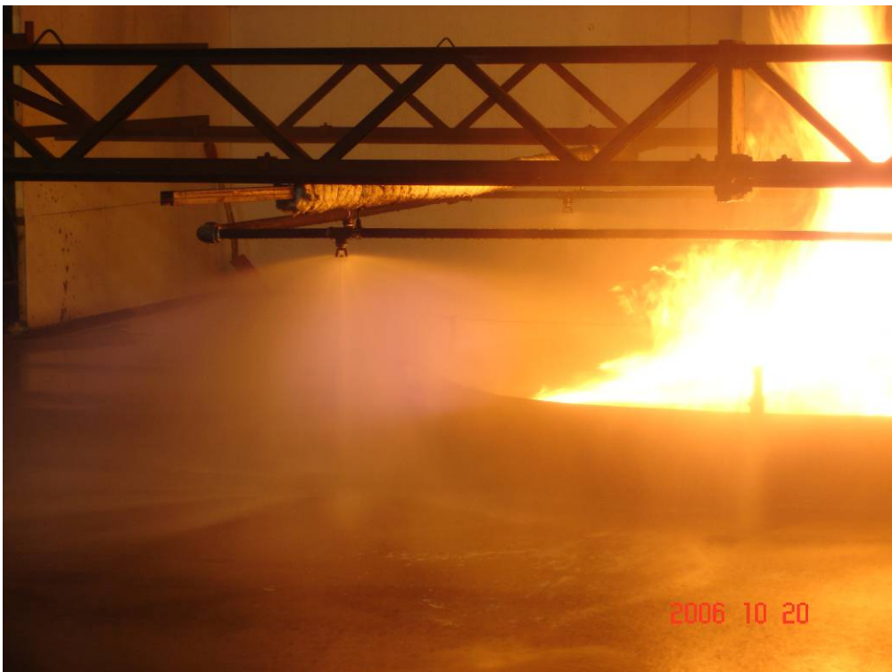
Photo 16 A close-up picture of the spray pattern of the nozzle type used for the tests where the distance to the fire was 0,55 m.
