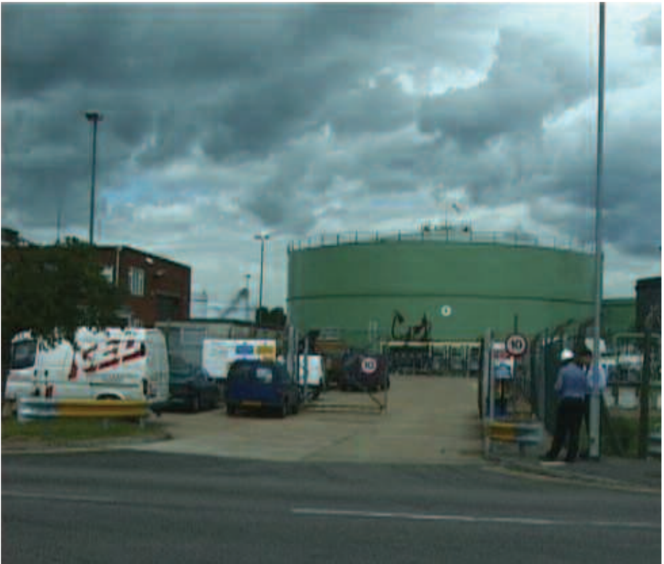
Figure 2 Looking into part of the Buncefield site before the incident. Note the ground vehicles, large storage tanks, and occupied buildings. To the right are manifolds that distributed fuel around the site
