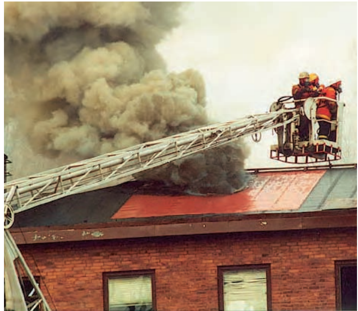
Figure 107. The smoke gases are streaming out from an attic fire.
