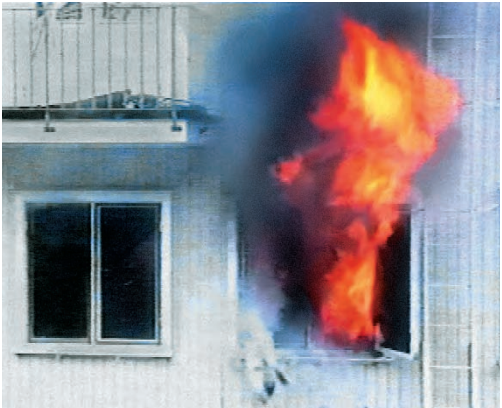
Figure 70. The fire is localised in the corner. There is still no indication that the fire's development is going to accelerate.
