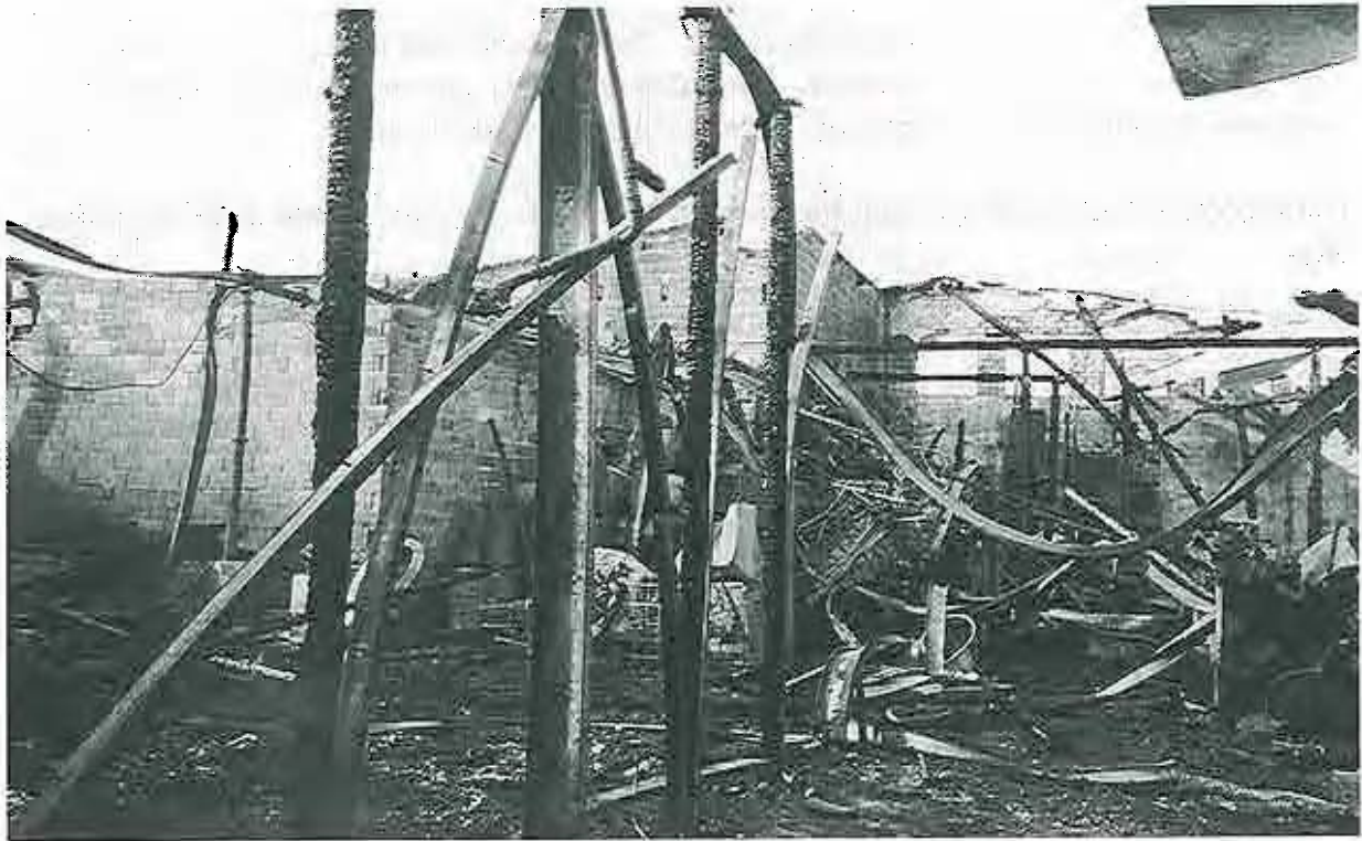
Fig. 4: The building in total ruin
