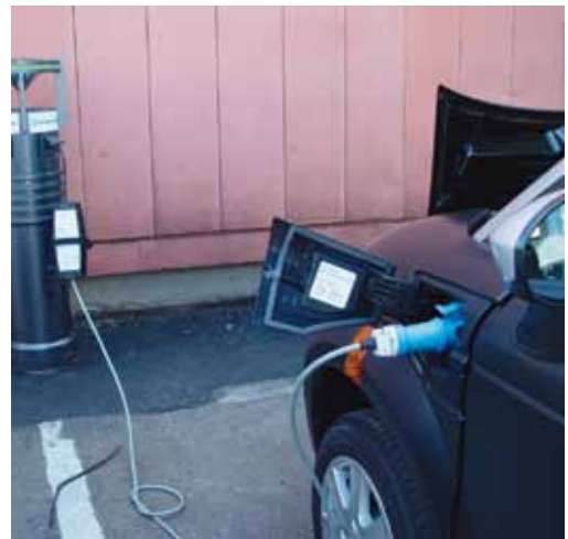
Electric car charging.
