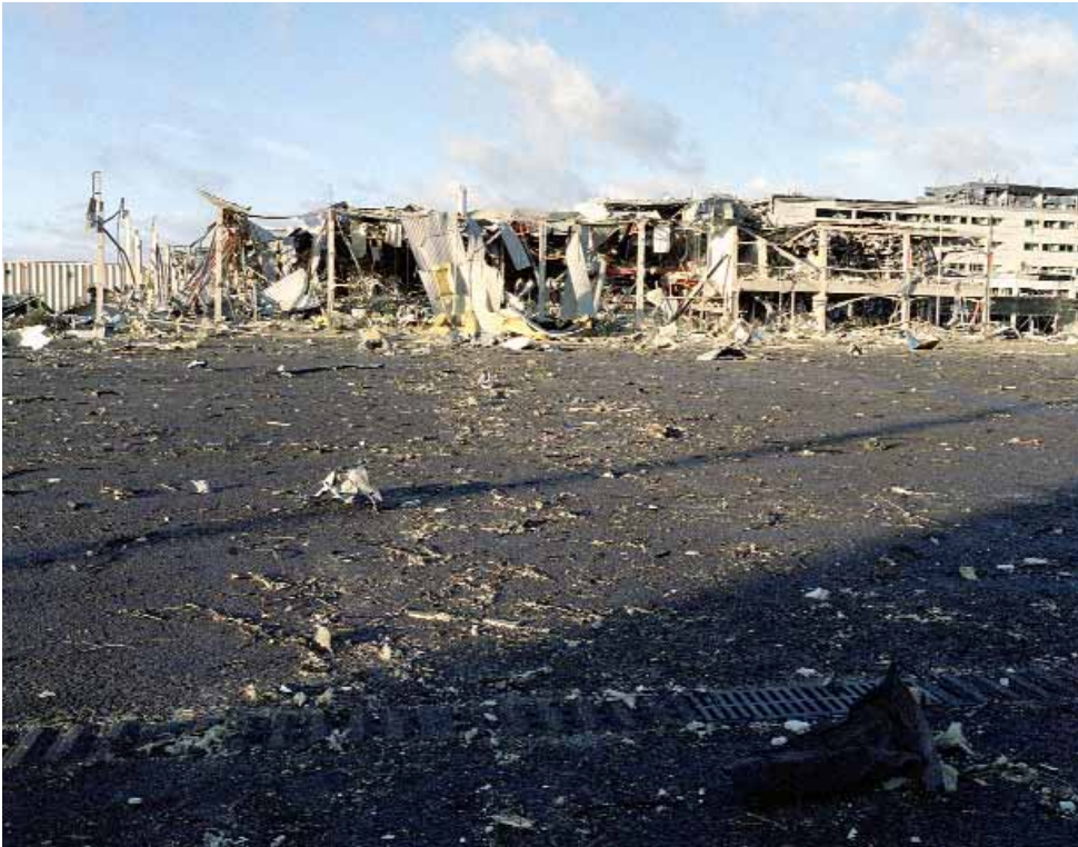
Figure 4 Fuji building looking north-west from the boundary with the Hertfordshire Oil Storage Ltd (HOSL) site
