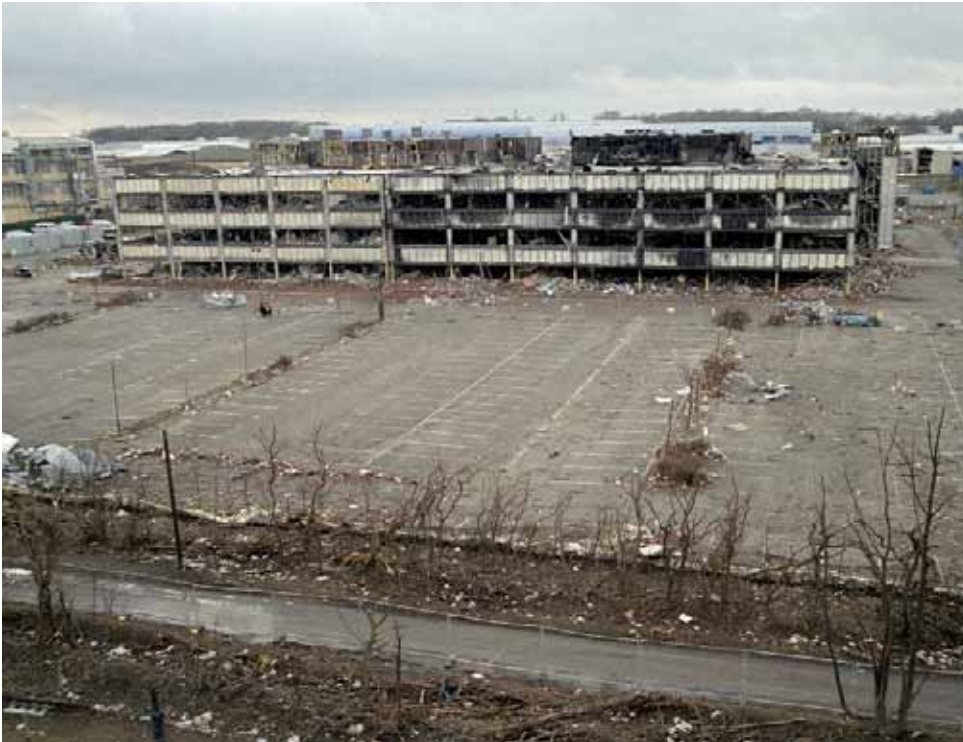
Figure 8 Looking west into Northgate building car park, from the position of Tank 912 (HOSL West)
