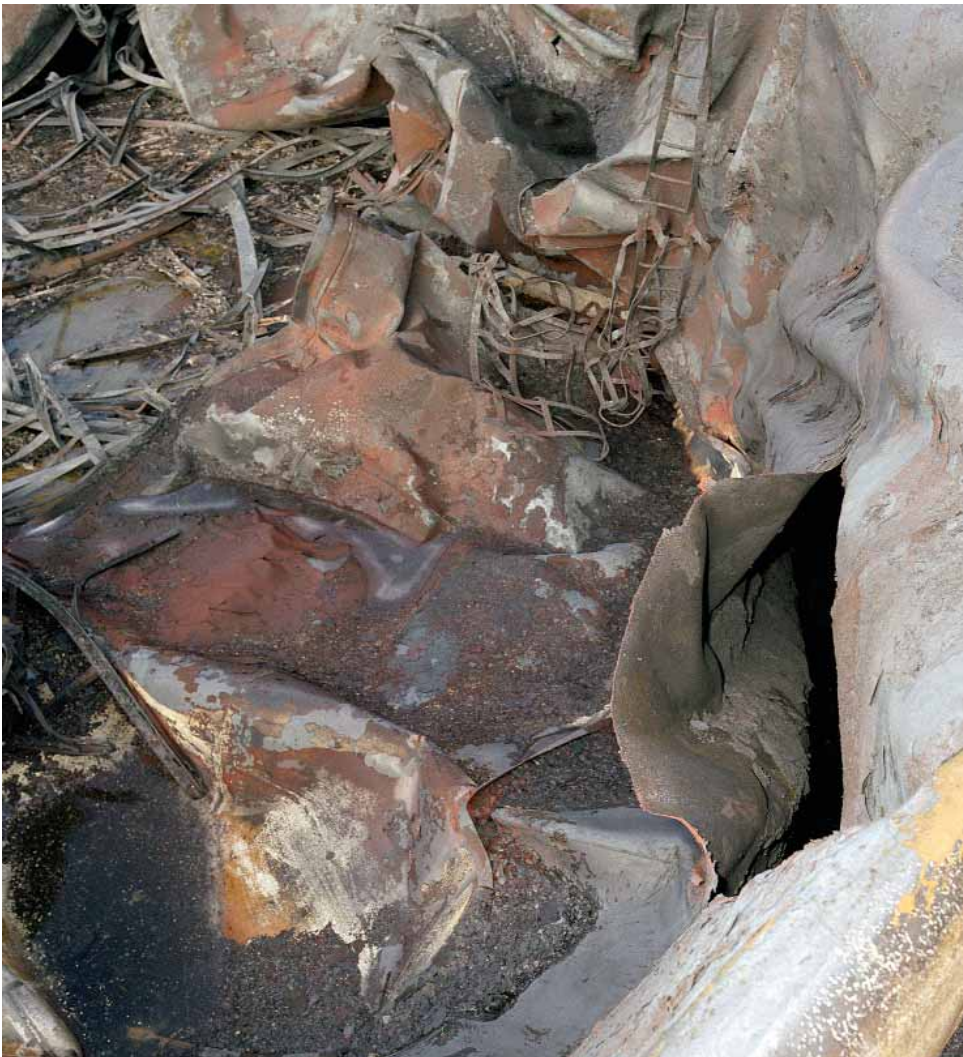
Figure 9 View into Tank 912
