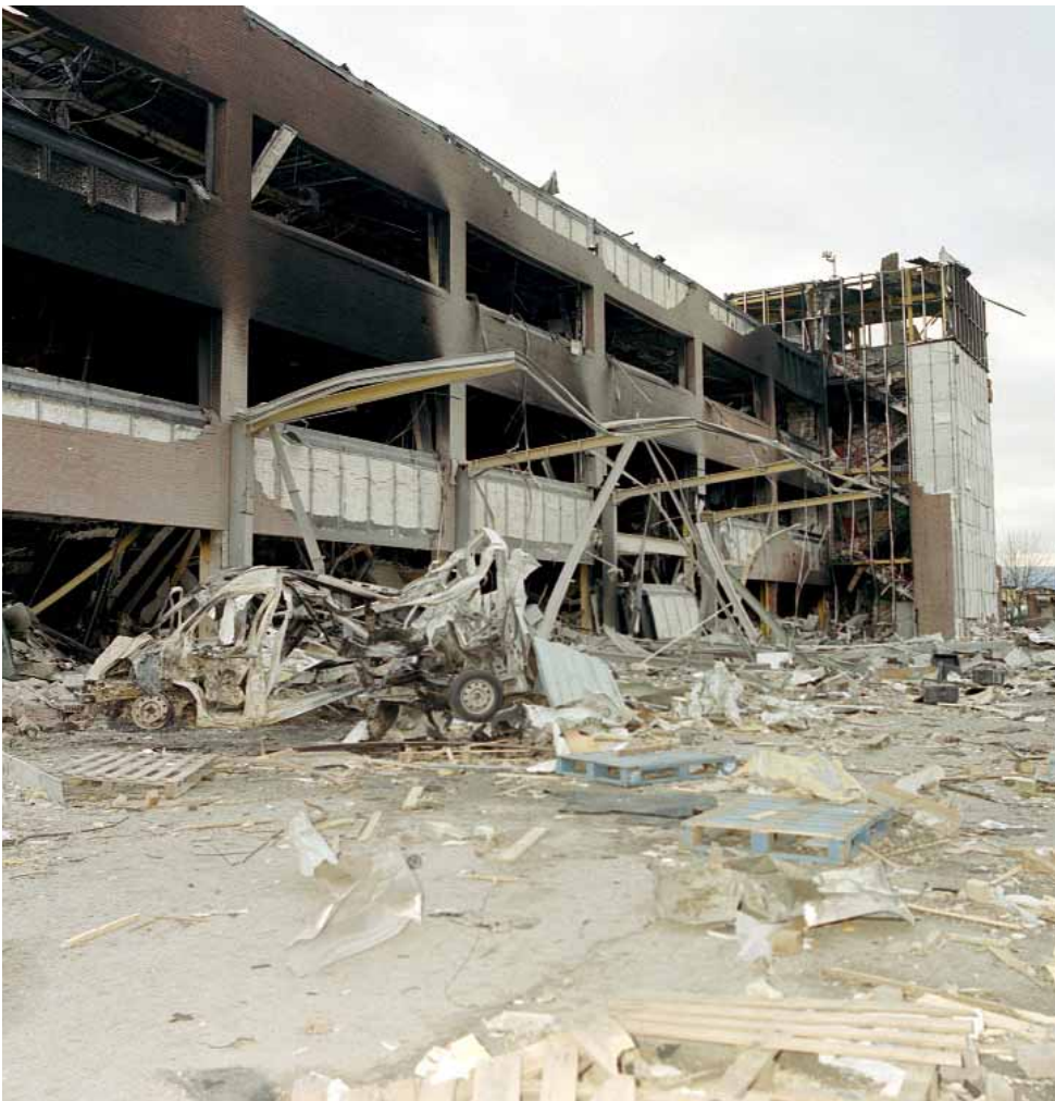
Figure 5 North side of the Northgate building
