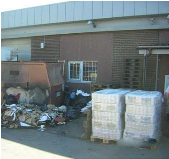
Brännbart material i alla former lagrades mot fasaden
