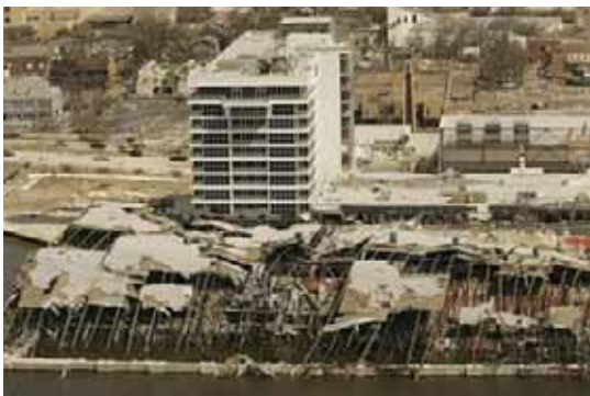
Biloxi: Hard Rock Casino partially destroyed
