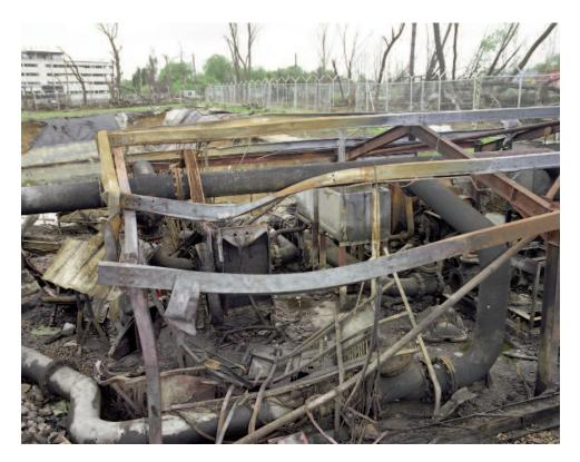
Figure 23 The remains of the fire pump house at the HOSL West site. The wall of bund A is approximately 5 m in front of this picture. The pump house is a prime candidate ignition source for the explosion at Buncefield
