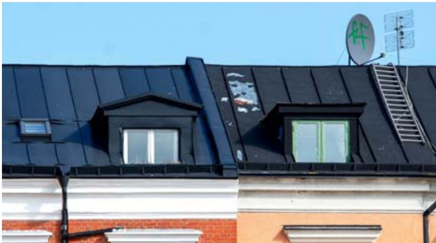
Example of a firewall that protrudes above the roof at the property boundary.
