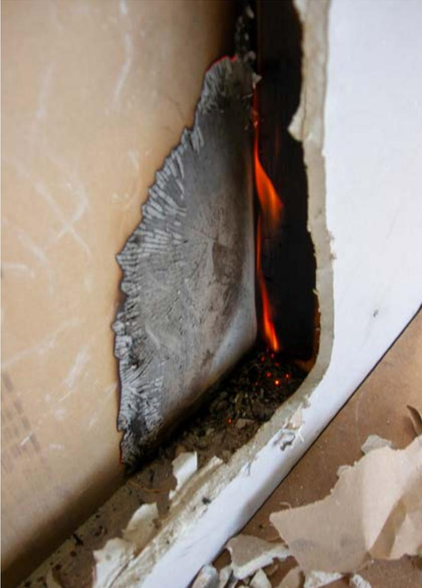
Smoldering fires inside structures are difficult to detect. For example, when a wall is broken open to access a smoldering fire, there is a risk of flame combustion occurring or the fire spreading as air is supplied. Photo: Stefan Svensson.
