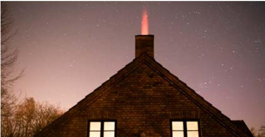
A chimney fire can produce flames that rise high above the chimney top. The risk of spreading to the building's structure is very high. Photo: Johnér Bildbyrå.
