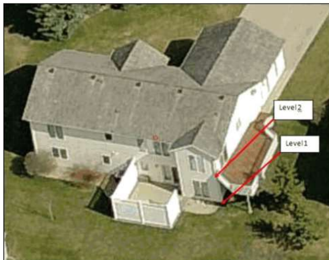
Figure 15. Number of stories for a single-family dwelling. Picture courtesy of pictometry. (FEMA, 2018)
