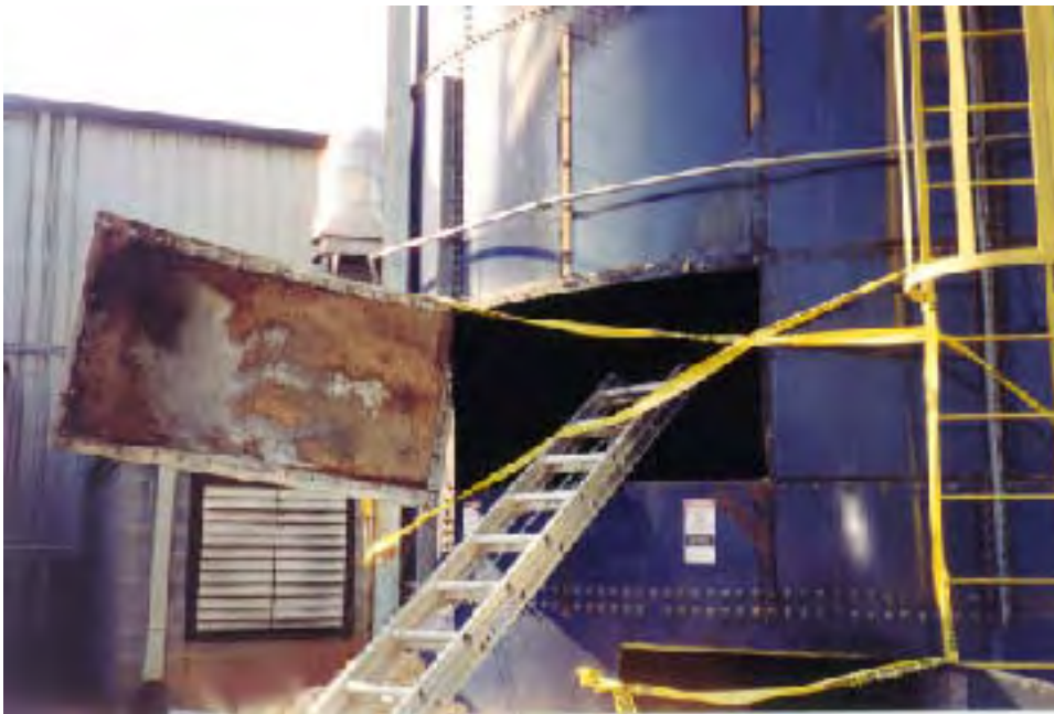
Photo 3. Access plate; area of origin of explosion
