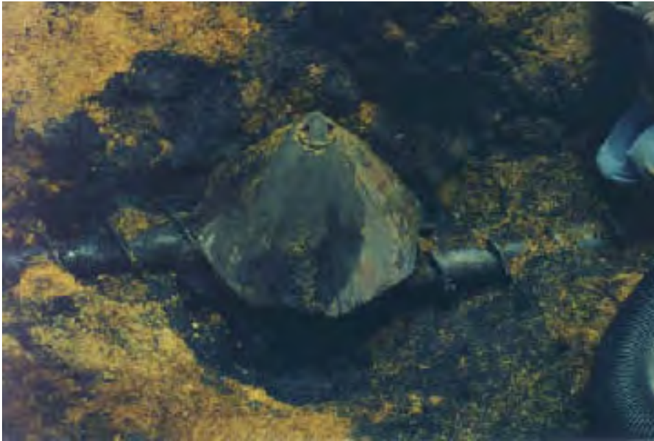
Photo 6. Auger gear box, covered by a shield suspected origin of fire
