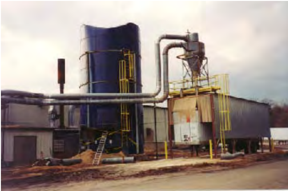
Photo 1. Silo with trailer shed to right and manufacturing facility in background
