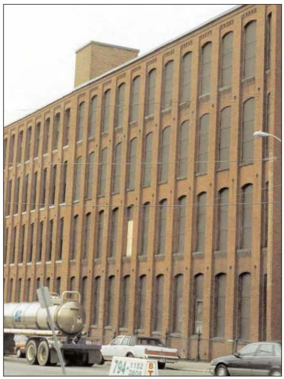
11. Windows once needed for natural light have been covered over, making visible fire location difficult. In addition, depending on the materials used, ventilation may be difficult.
