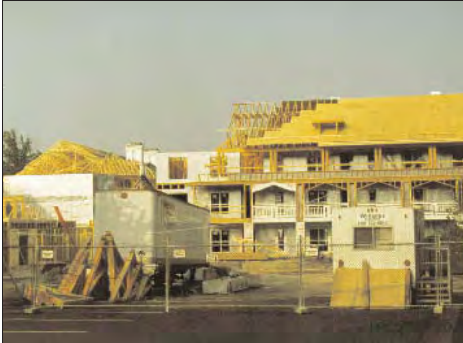
8. Reconstruction underway in Sector B, which is on the south side of the building. The exterior walkways were on this side of the wings.
