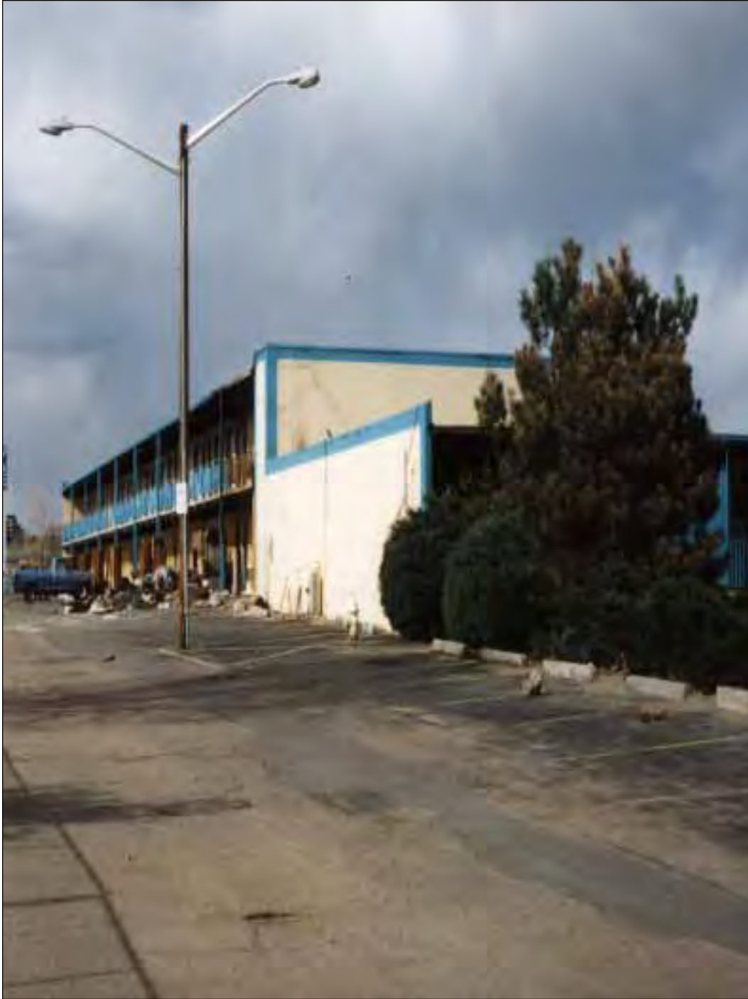
2. The west side of the property looking north. This is the 200 and 300 level guest rooms of the west wing and the end of the front wing. Engine 67 used the fire hydrant to the right of the light pole.
