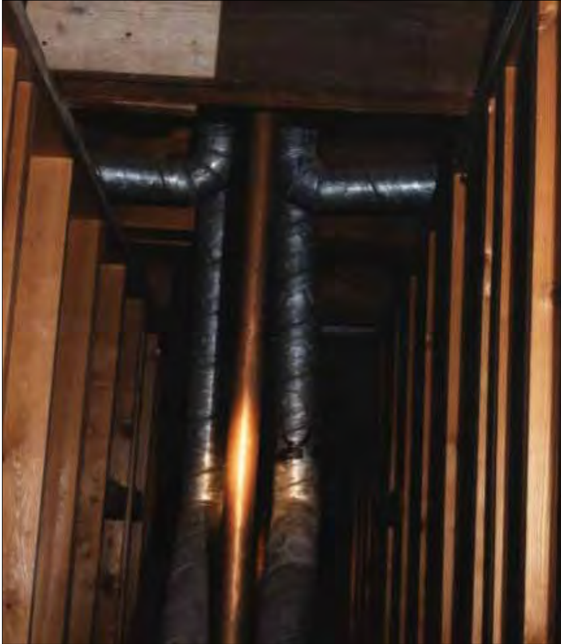
5. The interior of the utility chase between rooms showing the second floor wall construction and the wood beams supporting the roof.
