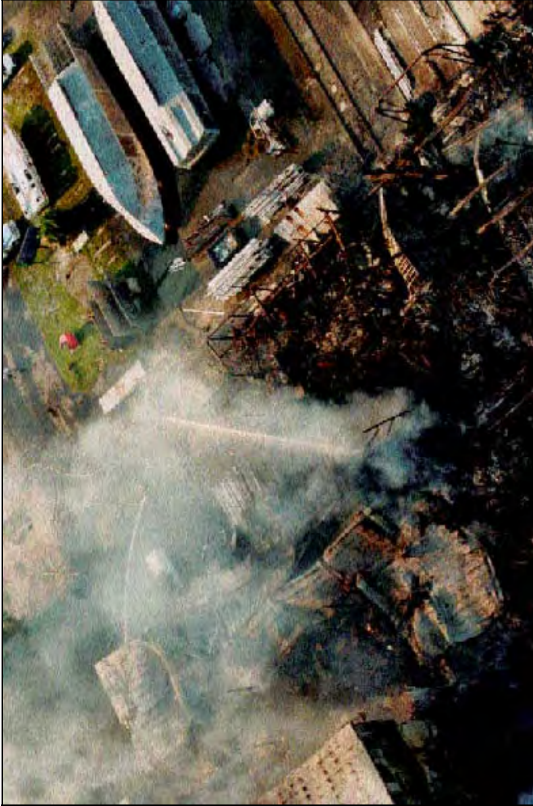
4. Aerial view of the south corner of the collapsed Manufacturing Building (Building A).
