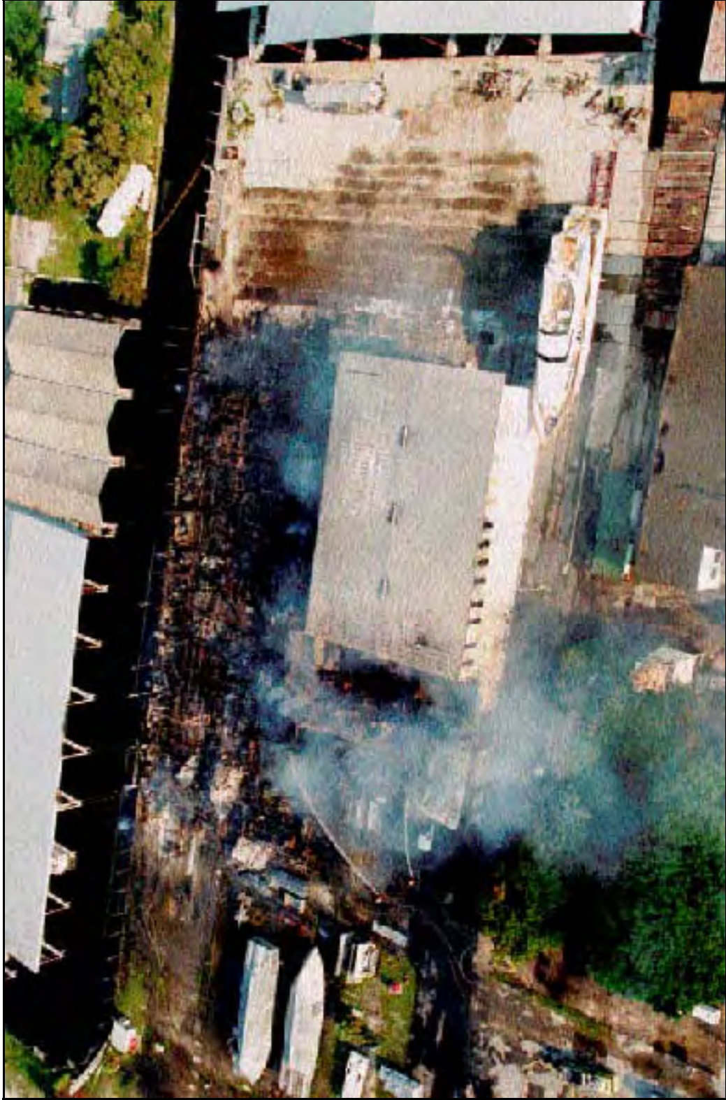
5. Aerial view of the fire scene, with the canal and neighboring covered boat slips (to the west) at top of photograph.
