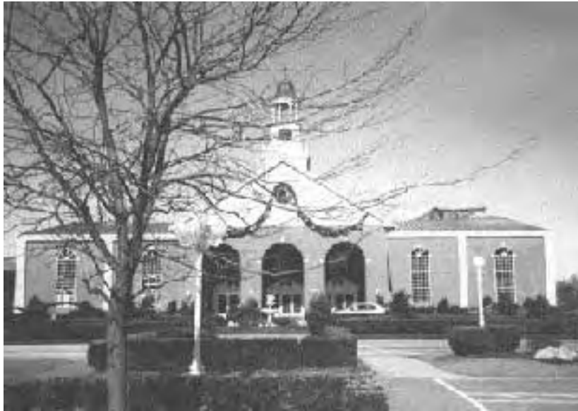
The front of the theater side one shows little damage because the fire wall between the auditorium and lobby held.
