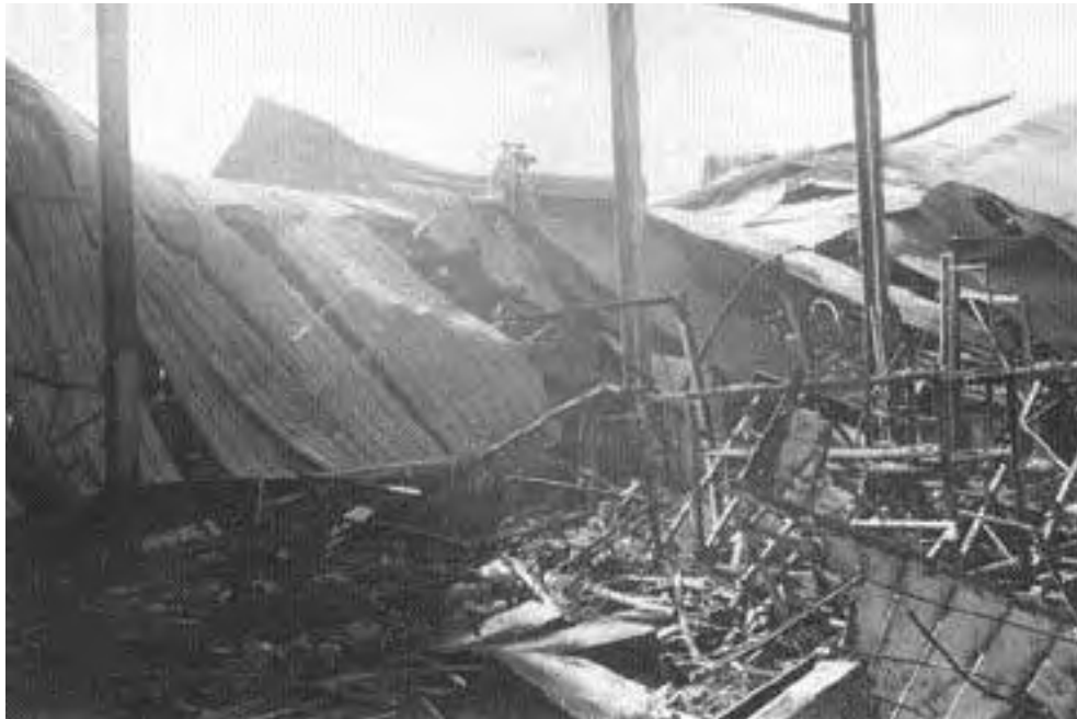
Shows the failure of the rear stage separation wall between the mechanical shops.
