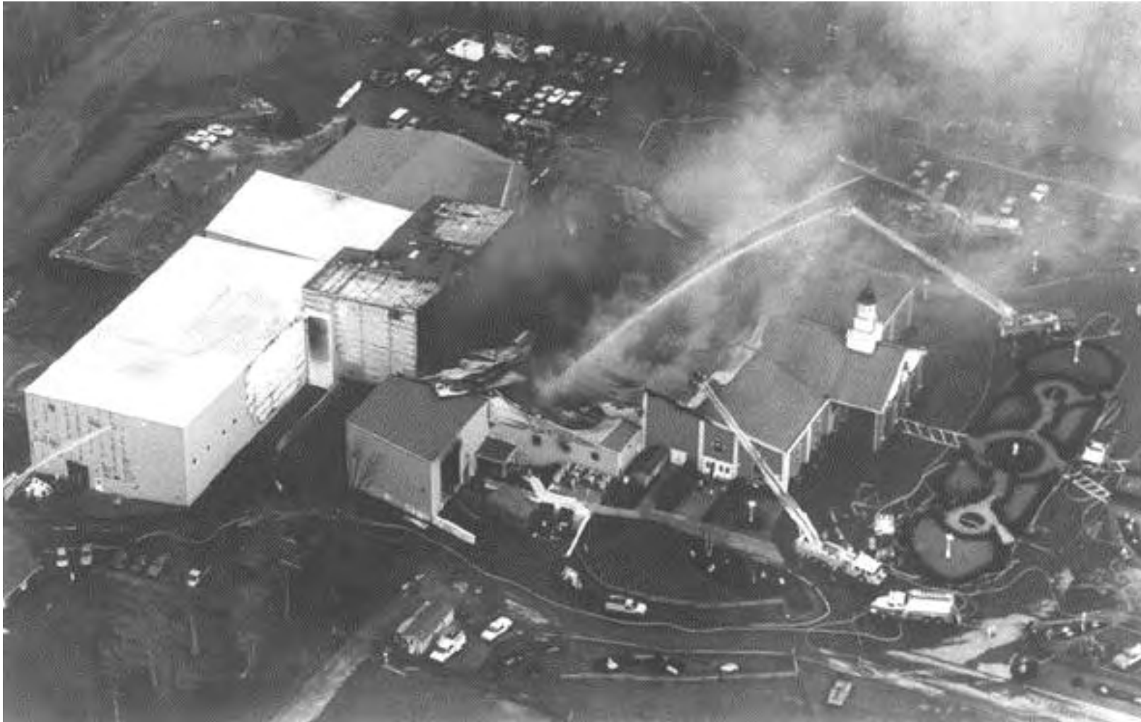
Aerial View One – shows the fire in progress after the auditorium roof collapsed. Note the four master streams and tanker relay hose lines.
