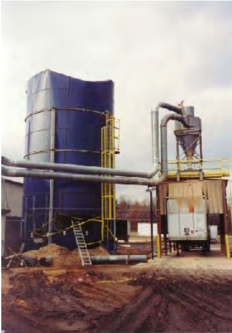
Damage to silo hatch at base. One firefighter blown onto roof of shed at right
