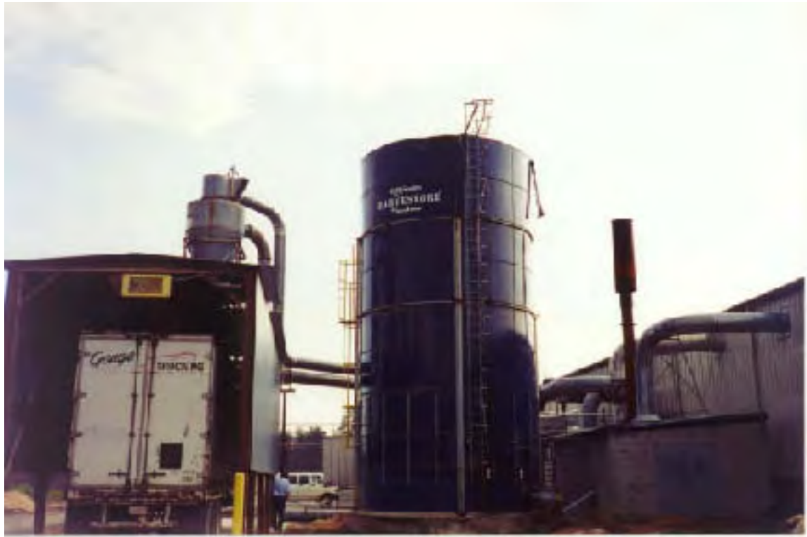
One portion of the roof traveled approximately 400' to the right
