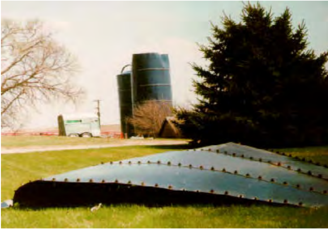
Travel distance of silo roof due to explosion
