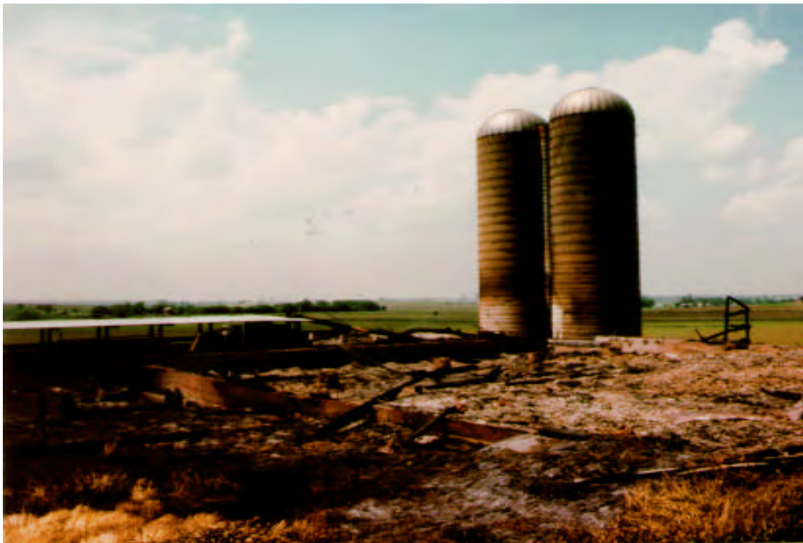
Fire originated in silo on right, extend to feed room dairy barn, cattle shed and feed
