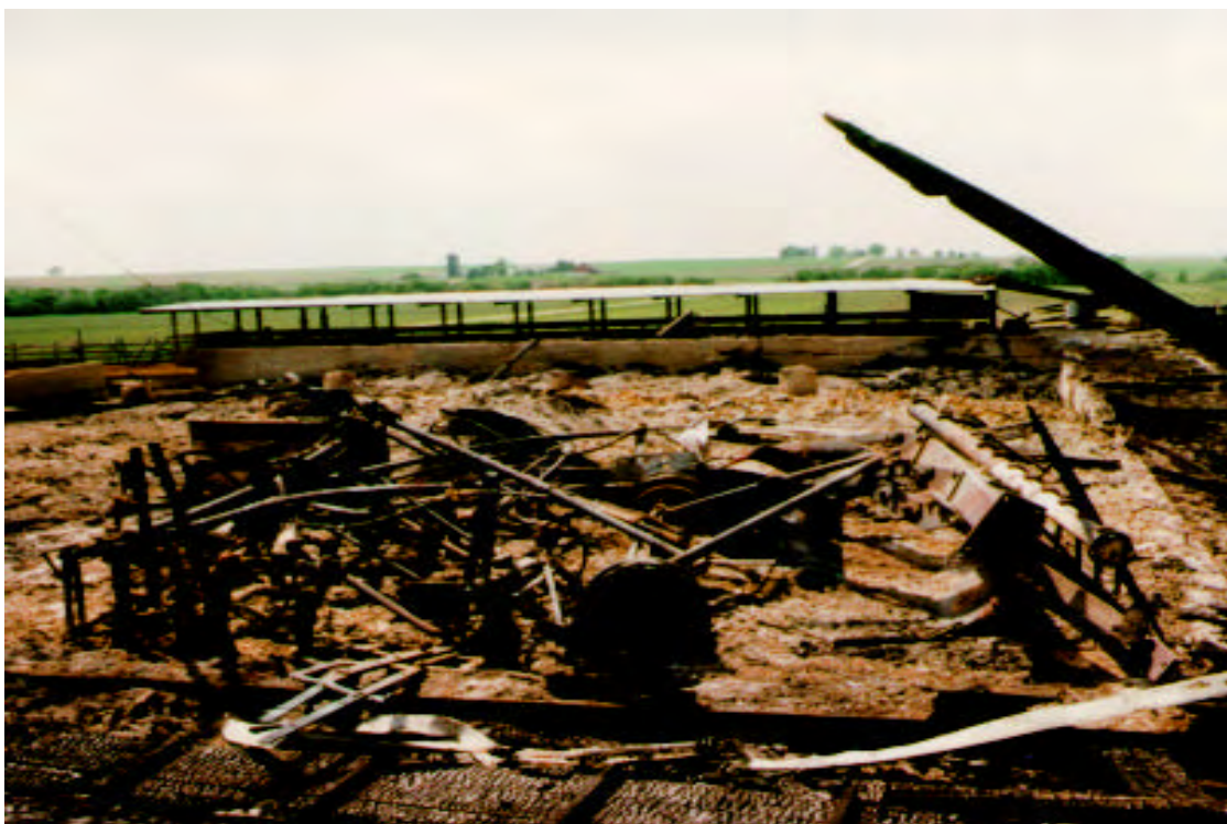
Destruction of farm buildings due to extension of spontaneous combustion - caused fire in silo
