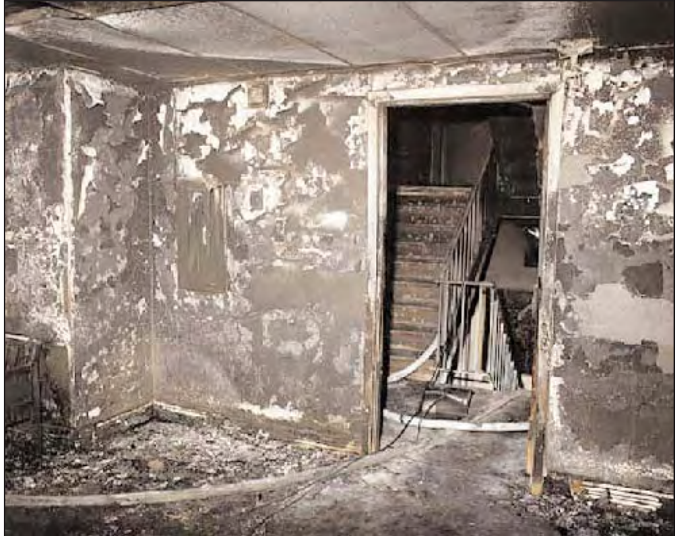
2. Doorway opening from SE stairway into office waiting area on second floor, adjacent to where investigators determined the fire originated.
