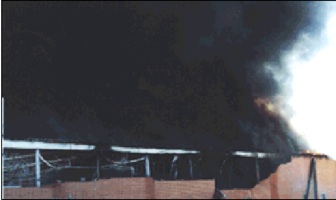
9. Conditions at the northwest corner of the building looking west from near Swift and Polk Streets. The outside post indicator valves (PIV's) and outside flow alarm bells for the sprinkler risers can be seen.
