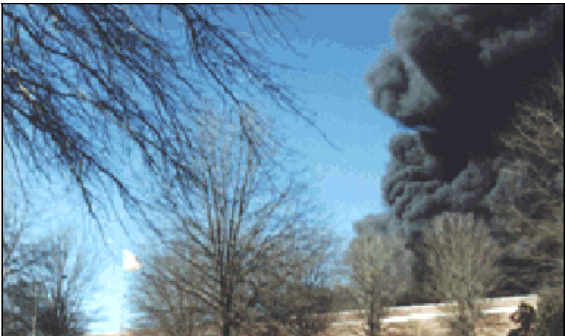
8. Conditions on the south side of the complex looking north from a position out from the northeast corner. At this point, the fire involves most of the 1972 addition.
