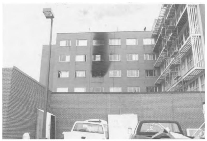
The first floor of the hospital extended out from the upper floors of the building, which blocked assess to the fourth floor windows by an aerial ladder. Firefighters used a ground ladder from the roof of the single story wing to rescue a patient from a window located two rooms to the left of the room of origin.
