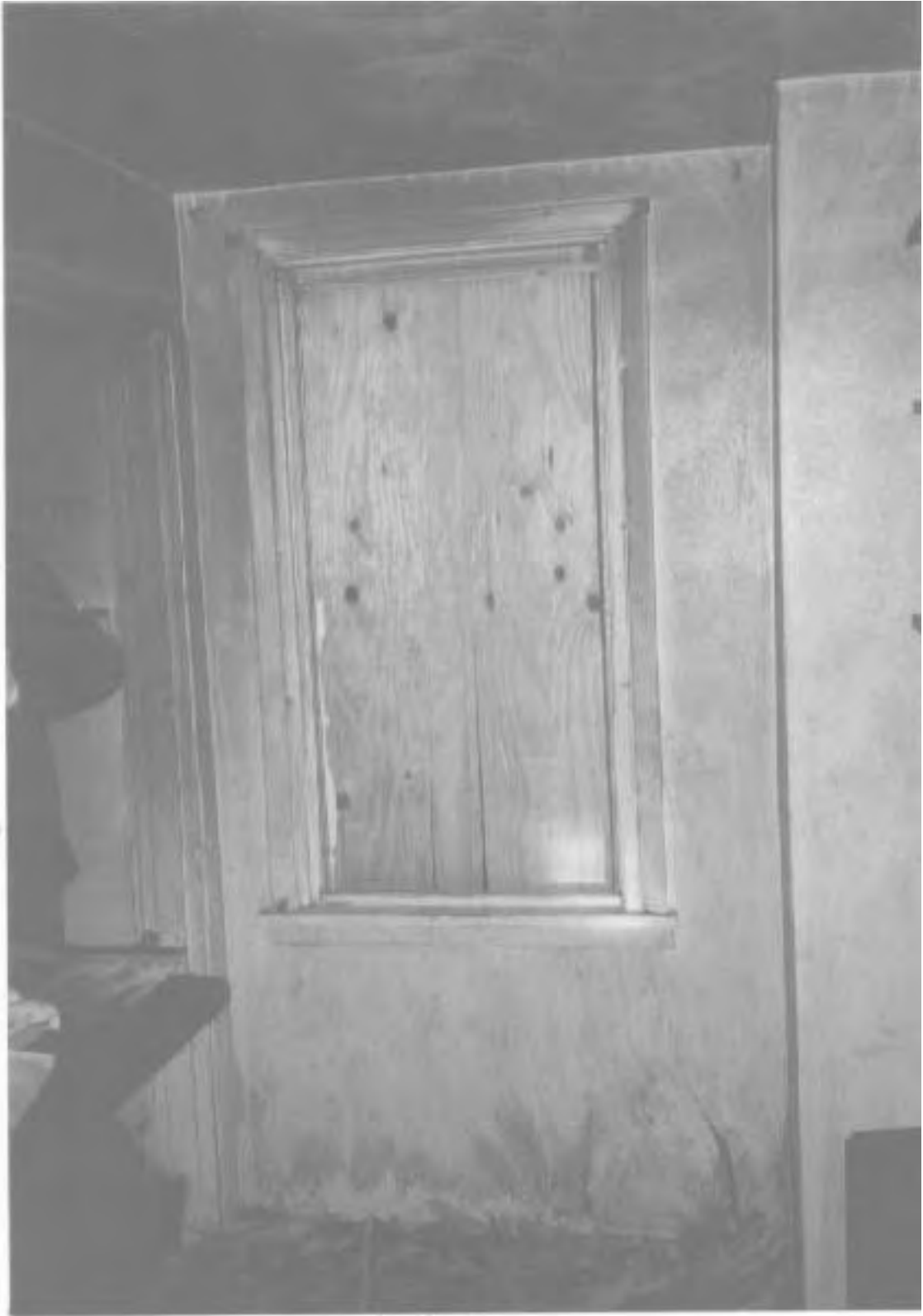
Inside view of window where firefighters were rescued.
