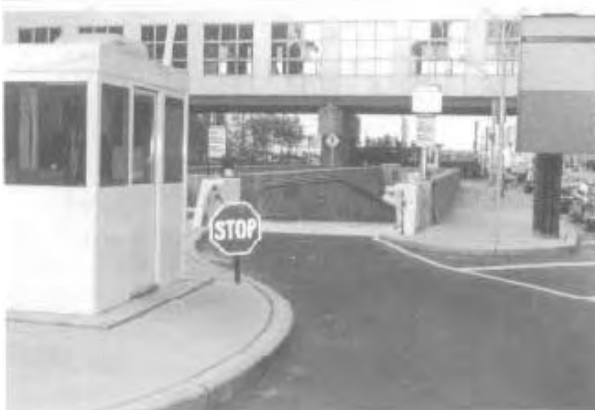
Controlling access to public buildings is a major concern for building management. After the incident, Port Authority, in addition to many security changes, installed substantial barriers to unauthorized vehicle access. The barrier, controlled by security personnel in the booth, folds down when the driver has been cleared to enter. (Photos courtesy of Port Authority Risk Management.)
