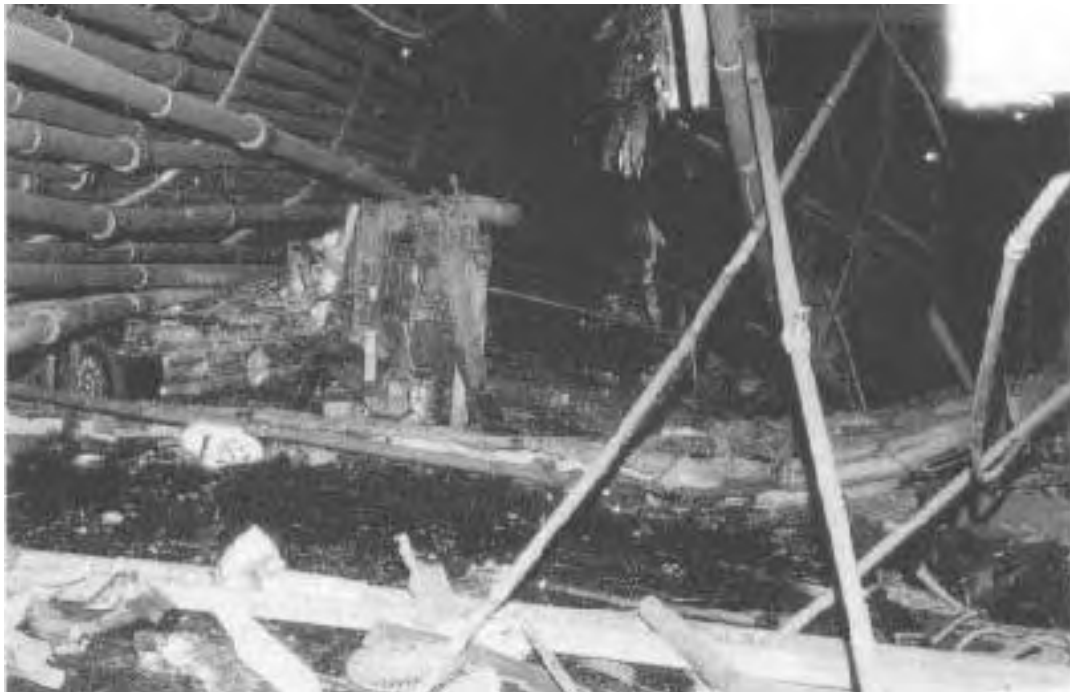
Building systems in the vicinity of the blast were destroyed. Here, twisted electrical conduit has landed on top of what was once a car. (Photo by FDNY Photo Unit.)
