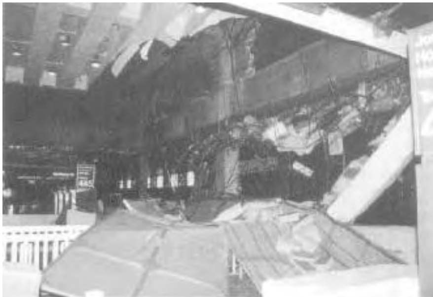
The explosion collapsed a portion of ceiling on the B-5 level onto a PATH train concourse. (Photos courtesy of Port Authority Risk Management.)
