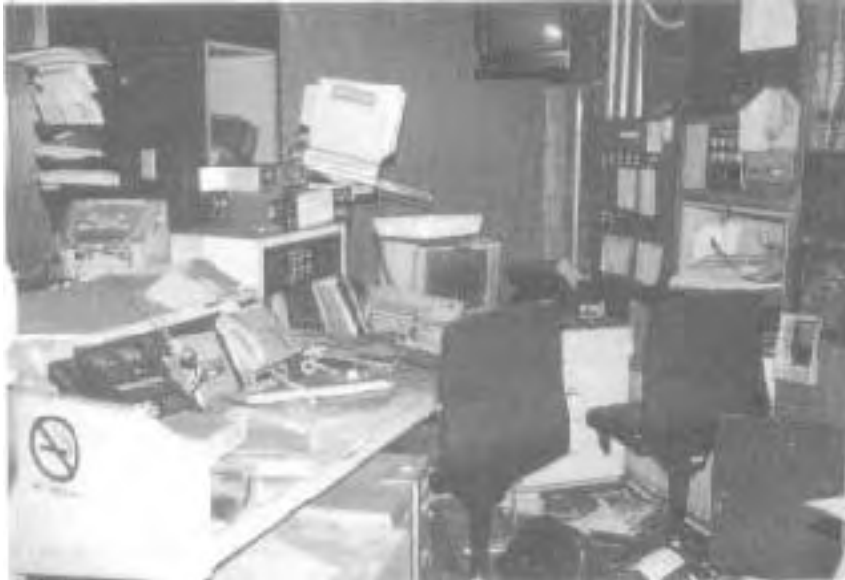
The Port Authority Command/Communications Center on the B-1 level, approximately 50 feet from the blast hole on that level, was damaged and communication with occupants in the towers was lost. (Photo courtesy of Port Authority Risk Management.)
