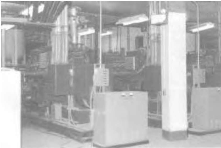
Emergency generators on the B-6 level. Cooling water lines for these units were ruptured by the blast, shutting down all emergency power. (Photo courtesy of Port Authority Risk Management.)
