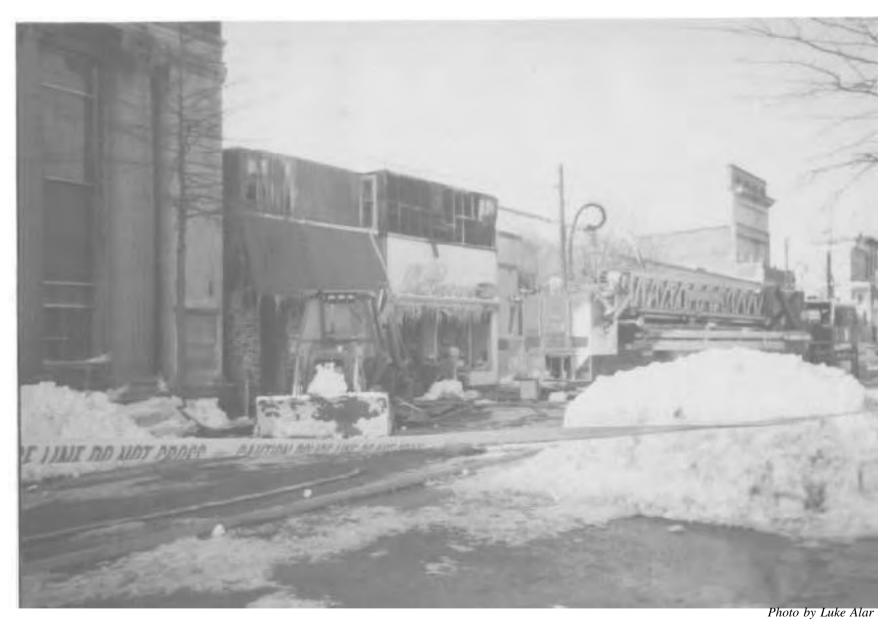
Approximately 16 hours after the fire, a backhoe is in front of the occupancy of fire origin to open an access to the coal bin under the sidewalk and provide access to the basement.
