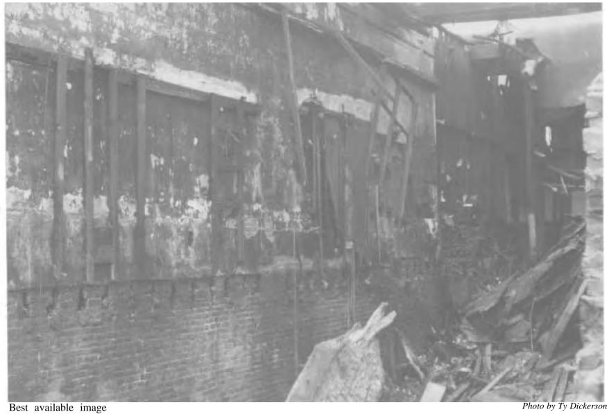
The wall of the front portion of the stationery store remains standing, although the interior is destroyed and the roof has collapsed.
