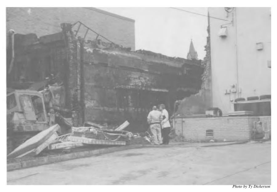
View of the area of fire origin and the area where the floor collapse occurred, after most of the debris has been removed. Indentations in the brick wall indicate where floor joists were supported.
