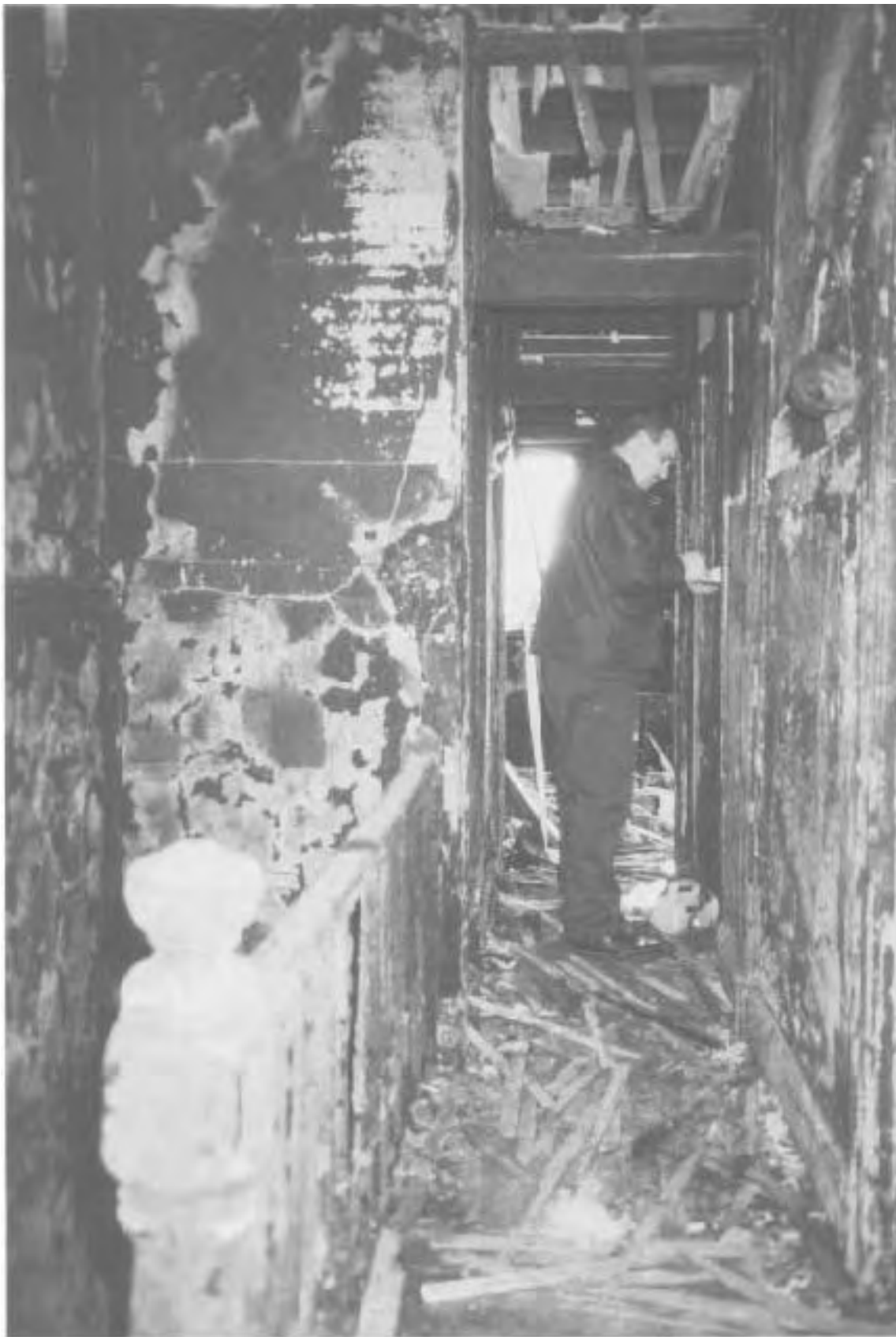
Second floor hallway looking toward front (master) bedroom. The burn pattern on the wall above the stairway opening is evidence of flame rollover from the intense fire in the dining room, kitchen, rear hallway, and bedroom below.
