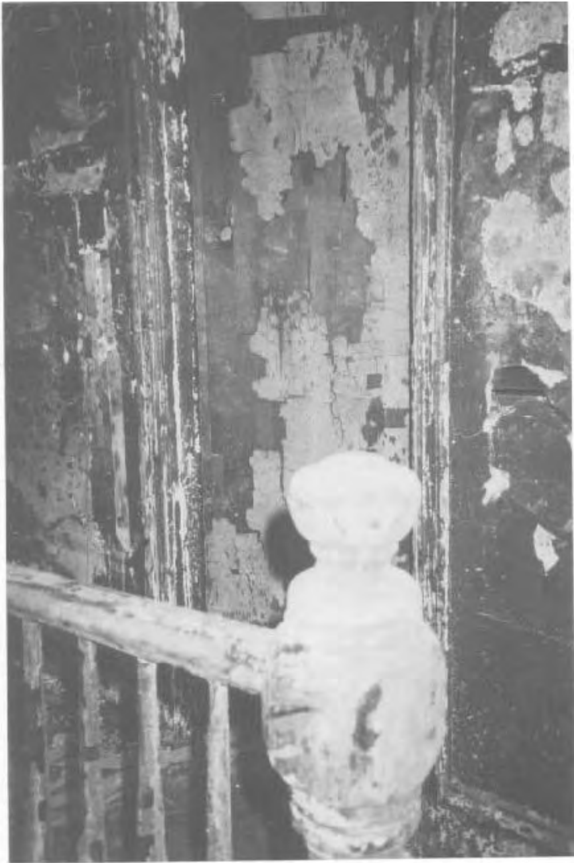
Rear doorway to second floor center bedroom. The homemade door is partially delaminated, explaining the irregular burn pattern.
