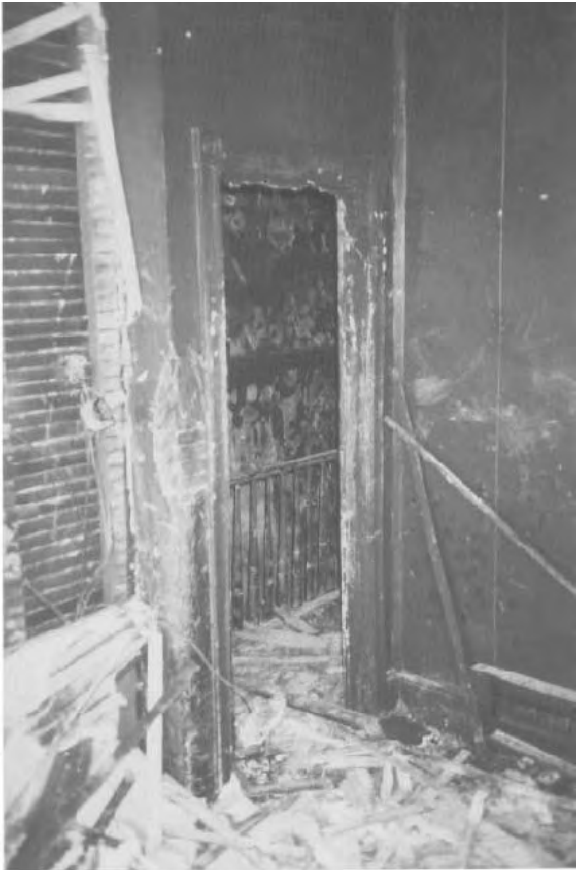
Entrance to second floor rear bedroom looking towards hallway. The door trim detail remains intact and heavy smoke residues stain the interior walls.
