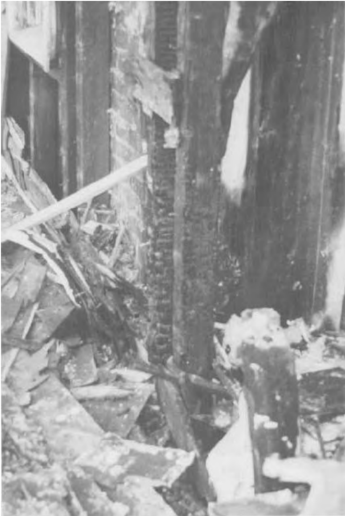
Charred stud in exterior wall of second floor rear bedroom. No firestopping was provided between the first and second floors. This is typical of balloon frame construction.
