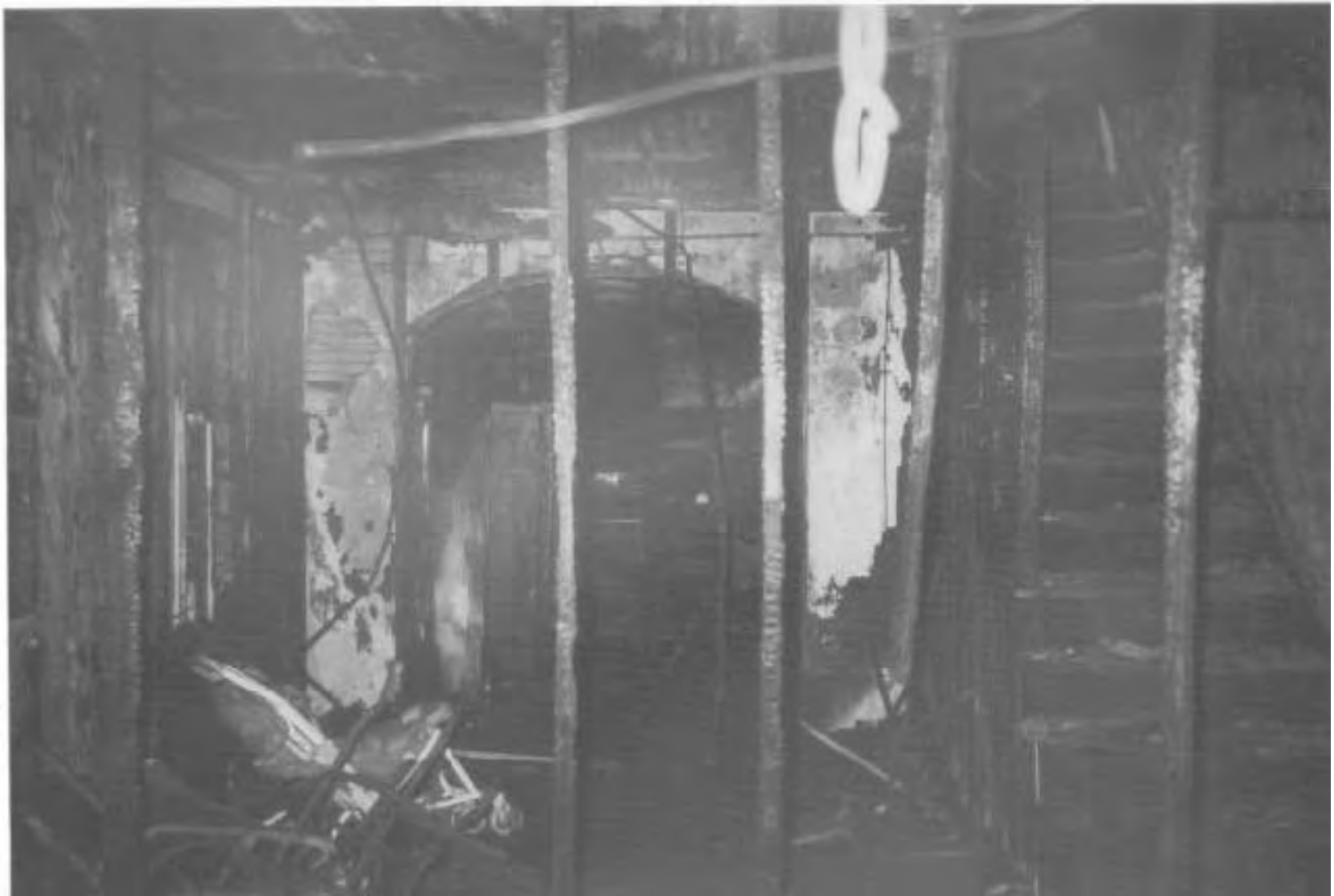
View from living room looking towards the rear of the house into the dining room. The unenclosed stairway was the primary path of heat and smoke travel to the second floor.
