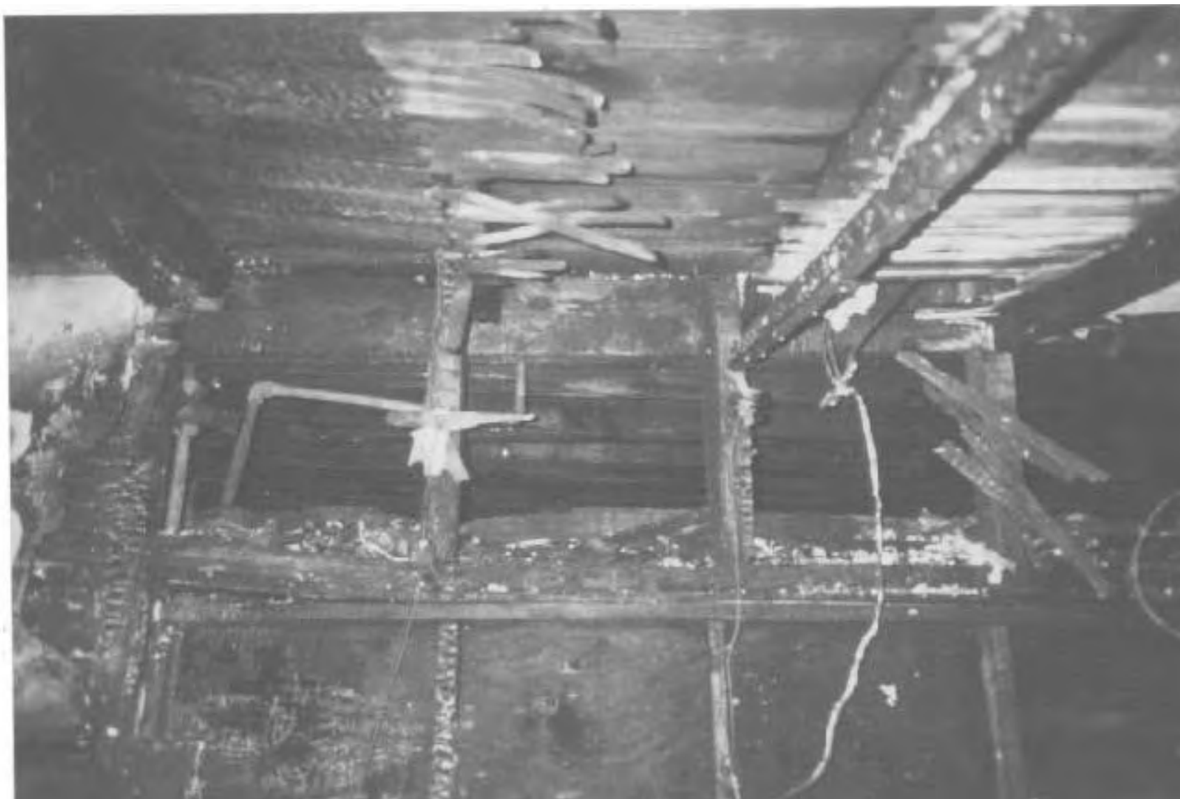
Wall and ceiling area above point of origin. Voids in the wall construction where the ceiling joists were attached permitted the fire to spread horizontally into the kitchen and vertically into the rear exterior wall of the bedroom above.
