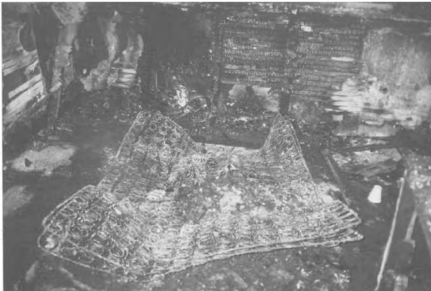
Point of origin in rear bedroom. The depressed floor area under the head of the bed was burned through to the crawl space below.
