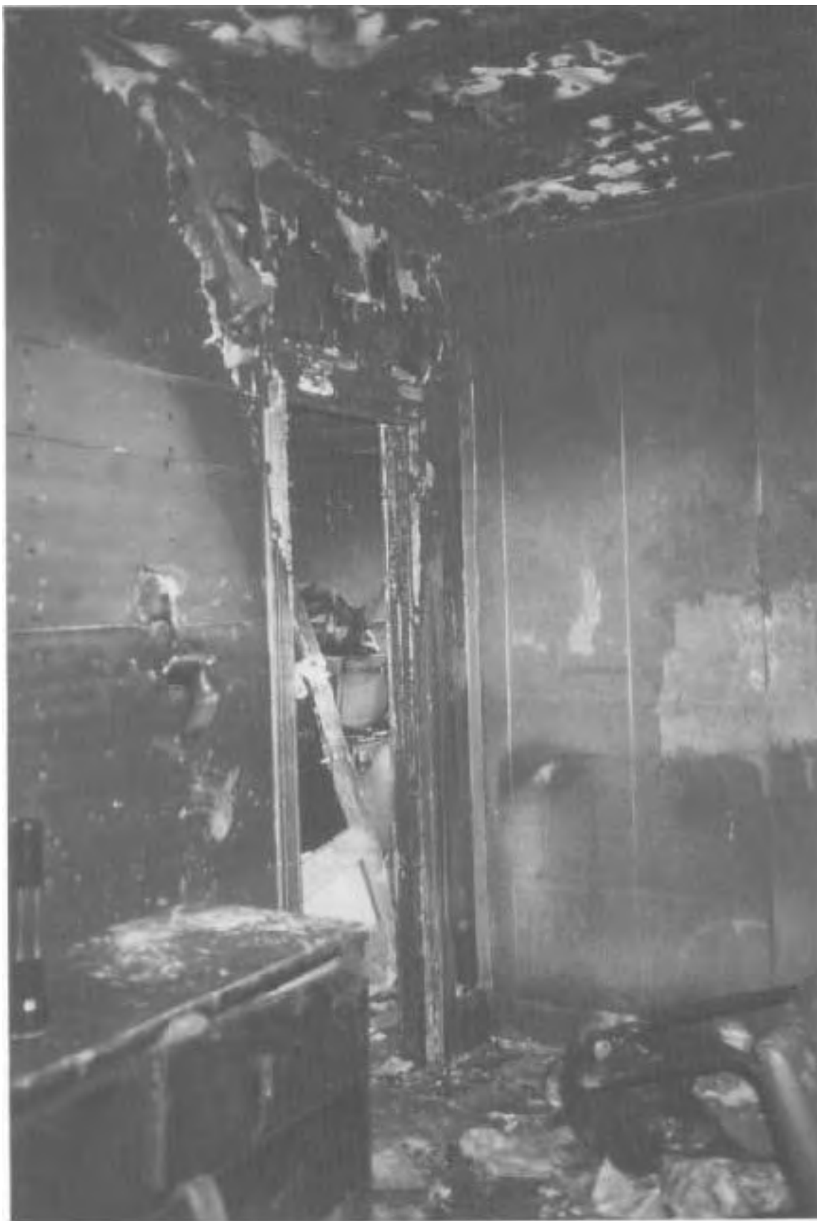
Thermal damage to wall and ceiling at top of front door opening to second floor center bedroom. This doorway was closed during the fire. However, convected heat and smoke from the fire below (see previous photograph) infiltrated the the doorway through air gap at the top of the door.
