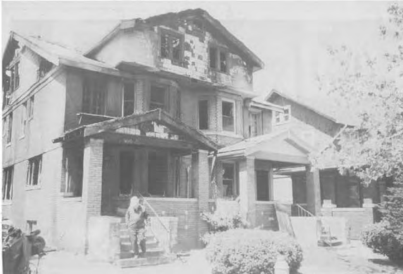
Exterior of 88-90 Pingree Street (structure faces south). Firefighters found fire showing from the first floor west and front, with heavy smoke showing from the second and third floors.
