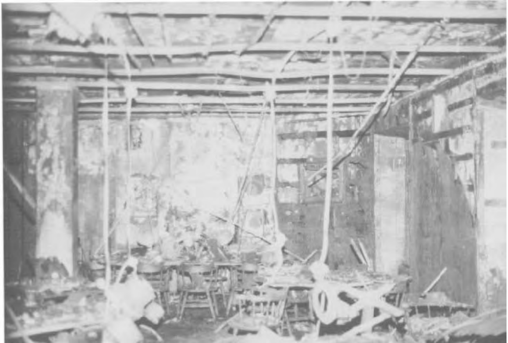
The inside of the McHale Room looking west. Shows the use of furring strips under the wall paneling. Much of the paneling at the remote west end of the room remains intact. Also note that the tops of the chair backs are only slightly blistered.
