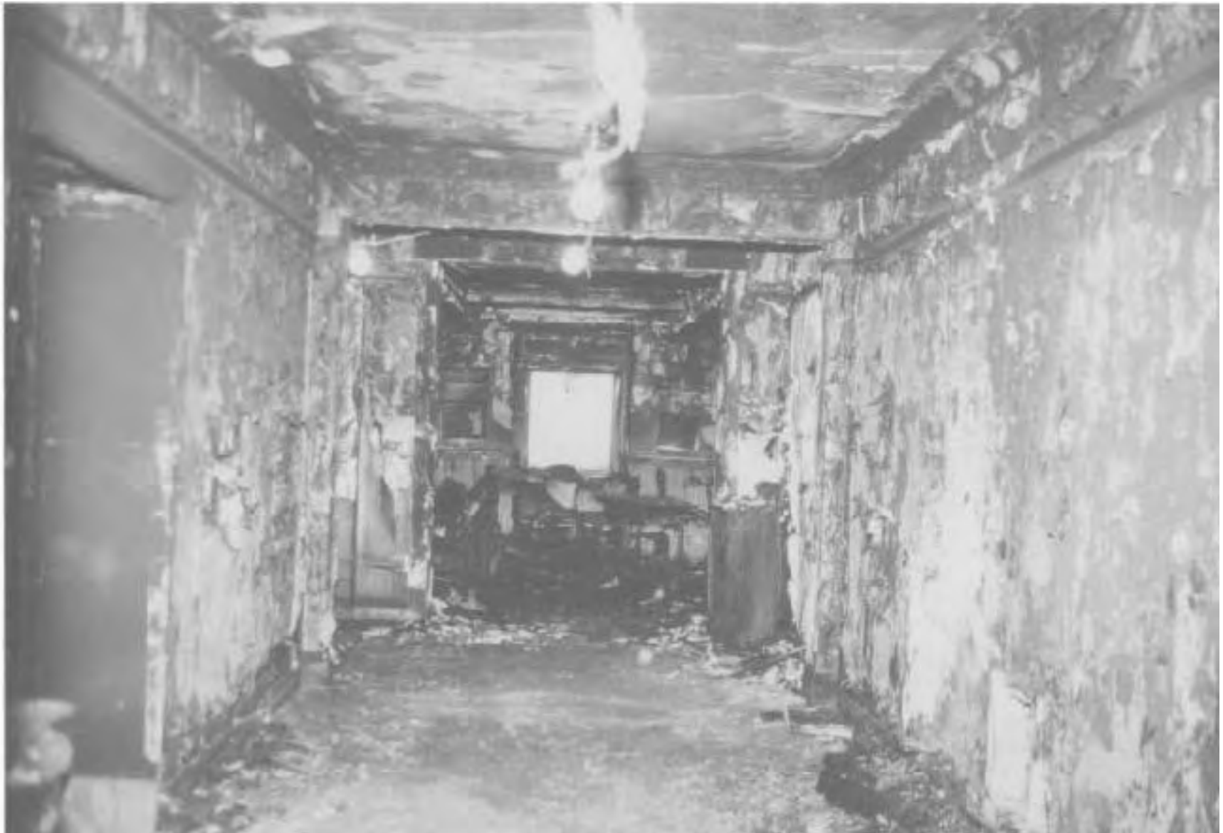
This view of the third floor corridor looking east toward the large dining room shows the extensive damage to combustible wallcoverings.
