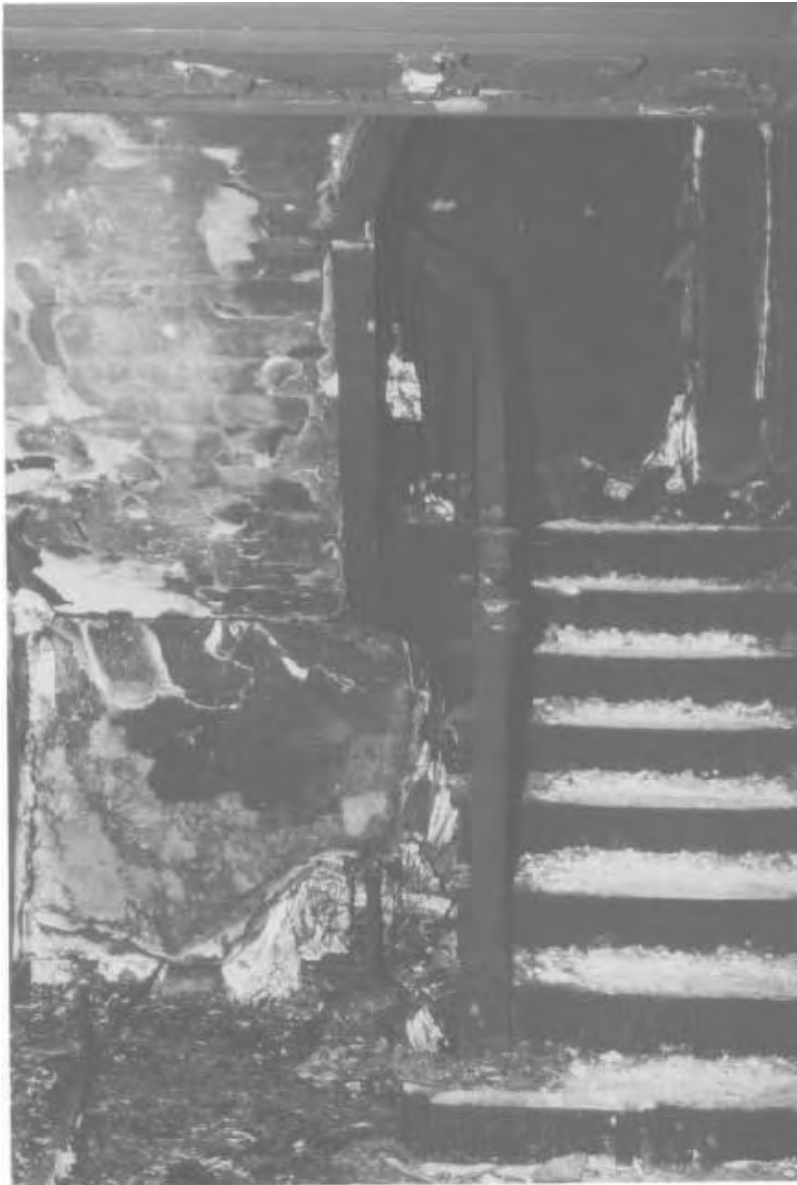
View of east stairway connecting third through ninth floors. This stairway was open on the third floor (shown here) and the fourth floor permitting the stairway to fill with smoke and the fire to spread vertically to the fourth floor.
