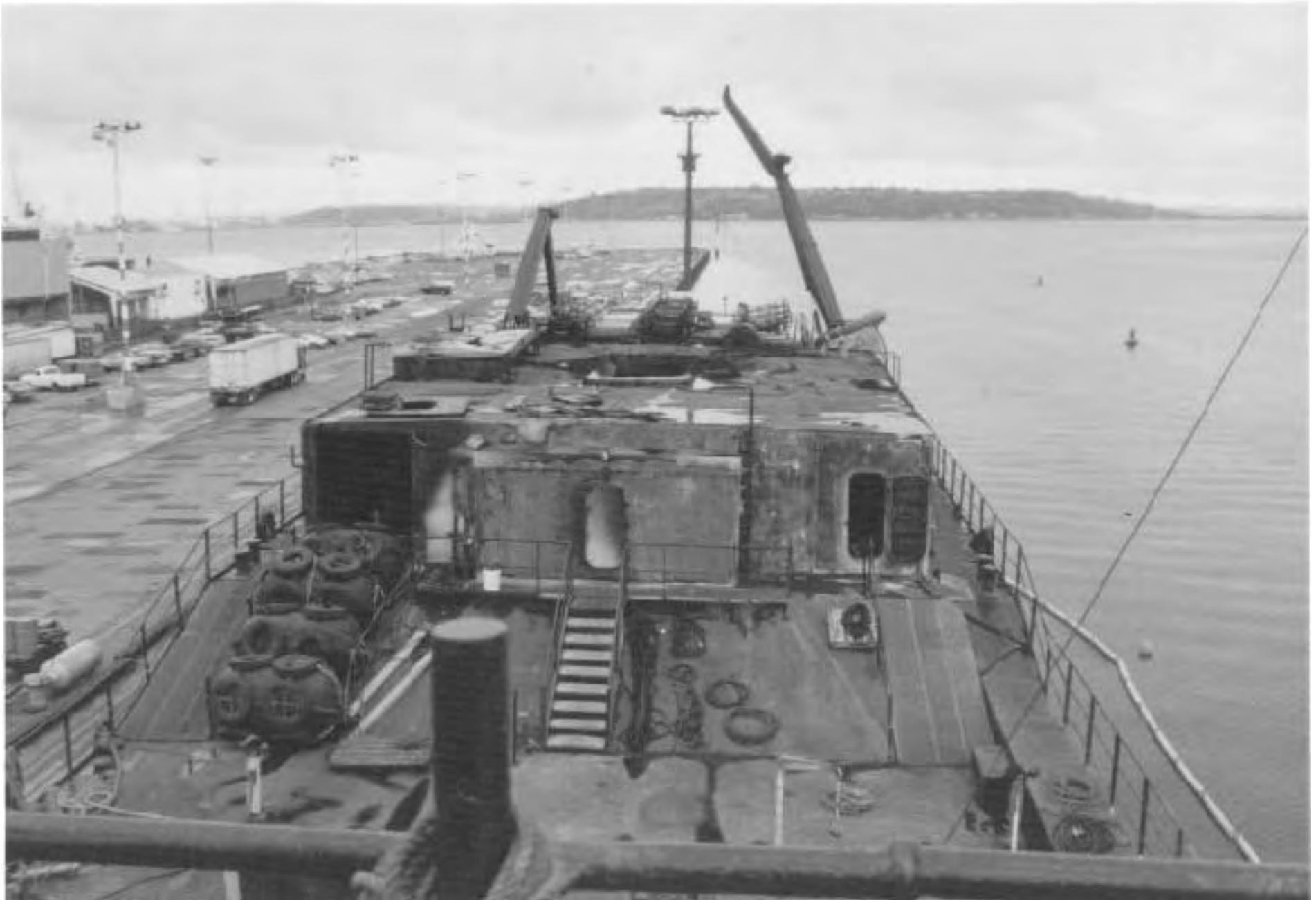
View from superstructure looking aft. Fish receiving house on deck. Major columns of fire and smoke came up from tween deck through square hole in the center of the "house." Another hatch and that hole had to be sealed.
