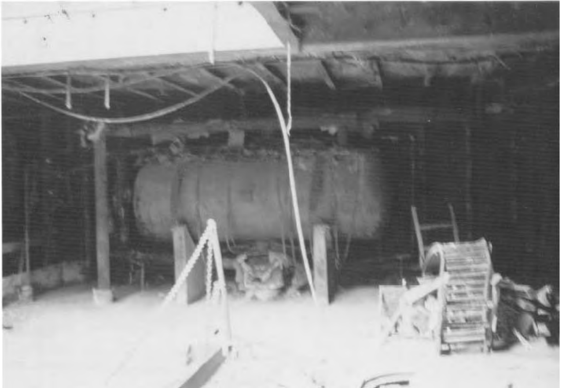
Ammonia tank in hold near fire origin.
