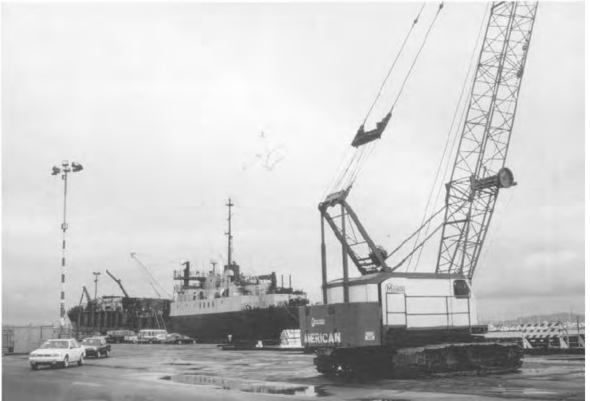
Crane used to lift steel plates on board.
