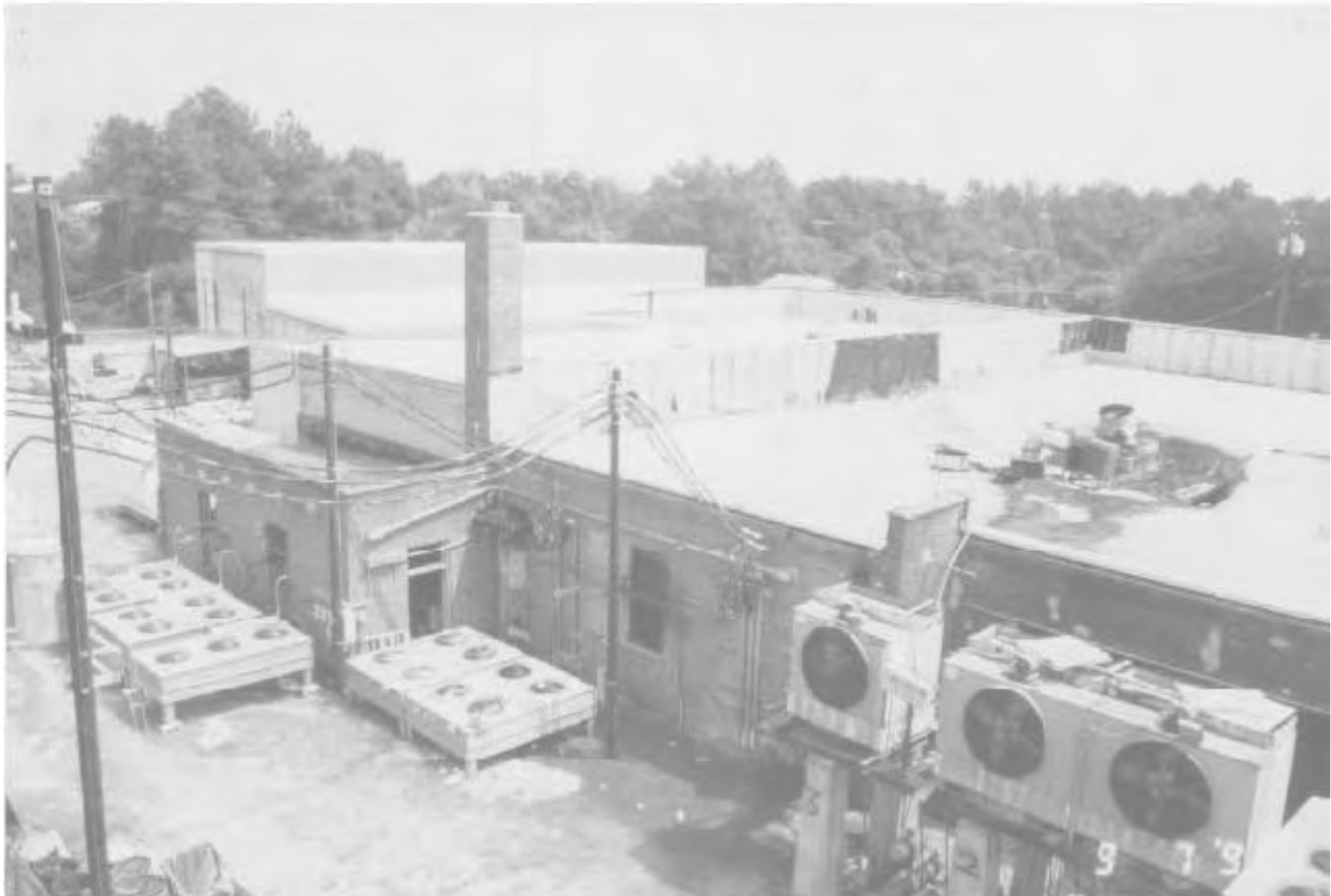
A view from the aerial ladder from the west side looking to the northeast. The roof collapse can be seen on the right, refrigeration compressor equipment is seen on the ground in the lower left.
