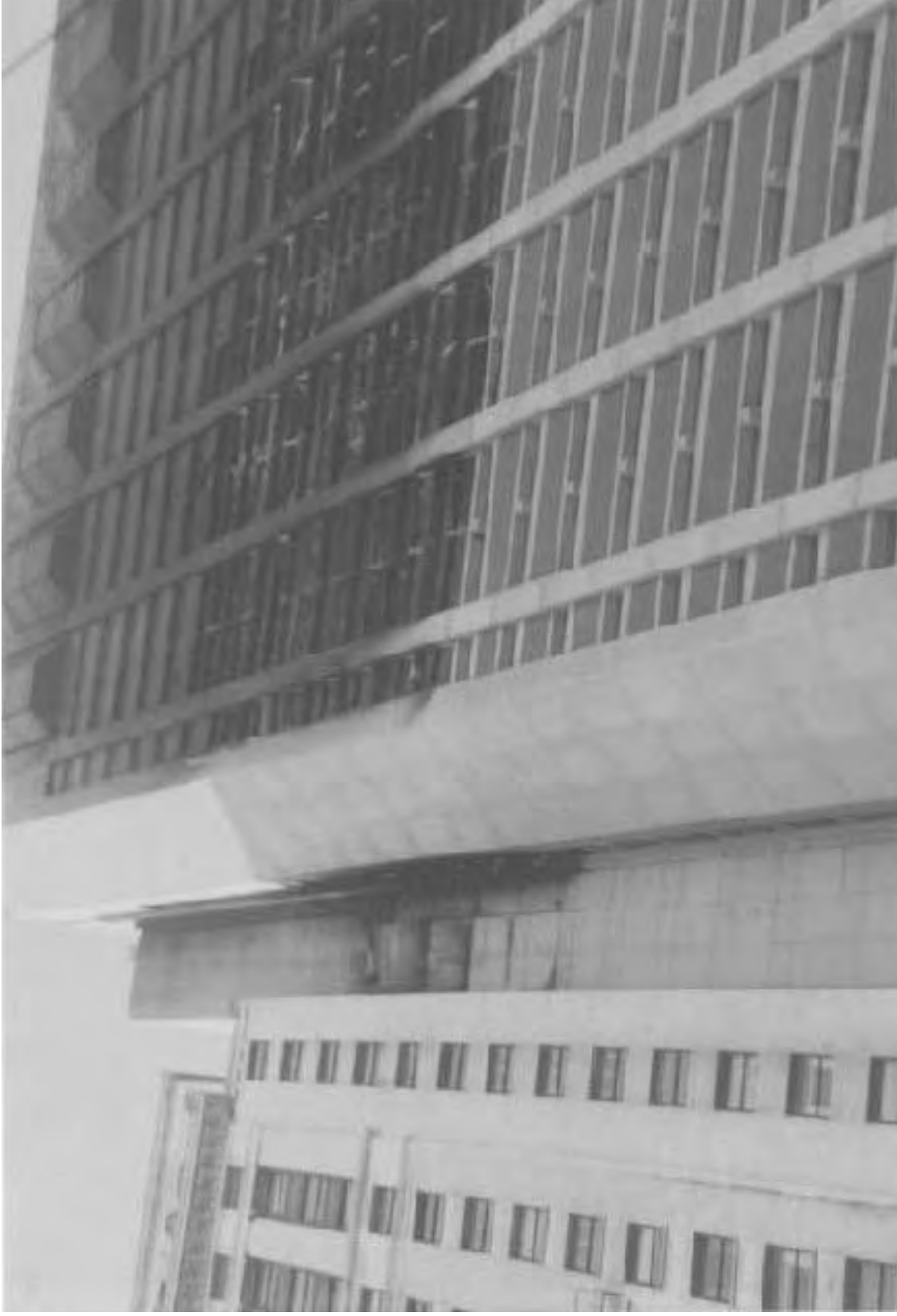
This stairway connected the One Meridian Plaza Building with the adjacent office building.
