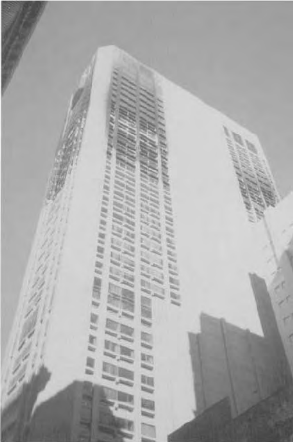
Exterior view of south side of building.
