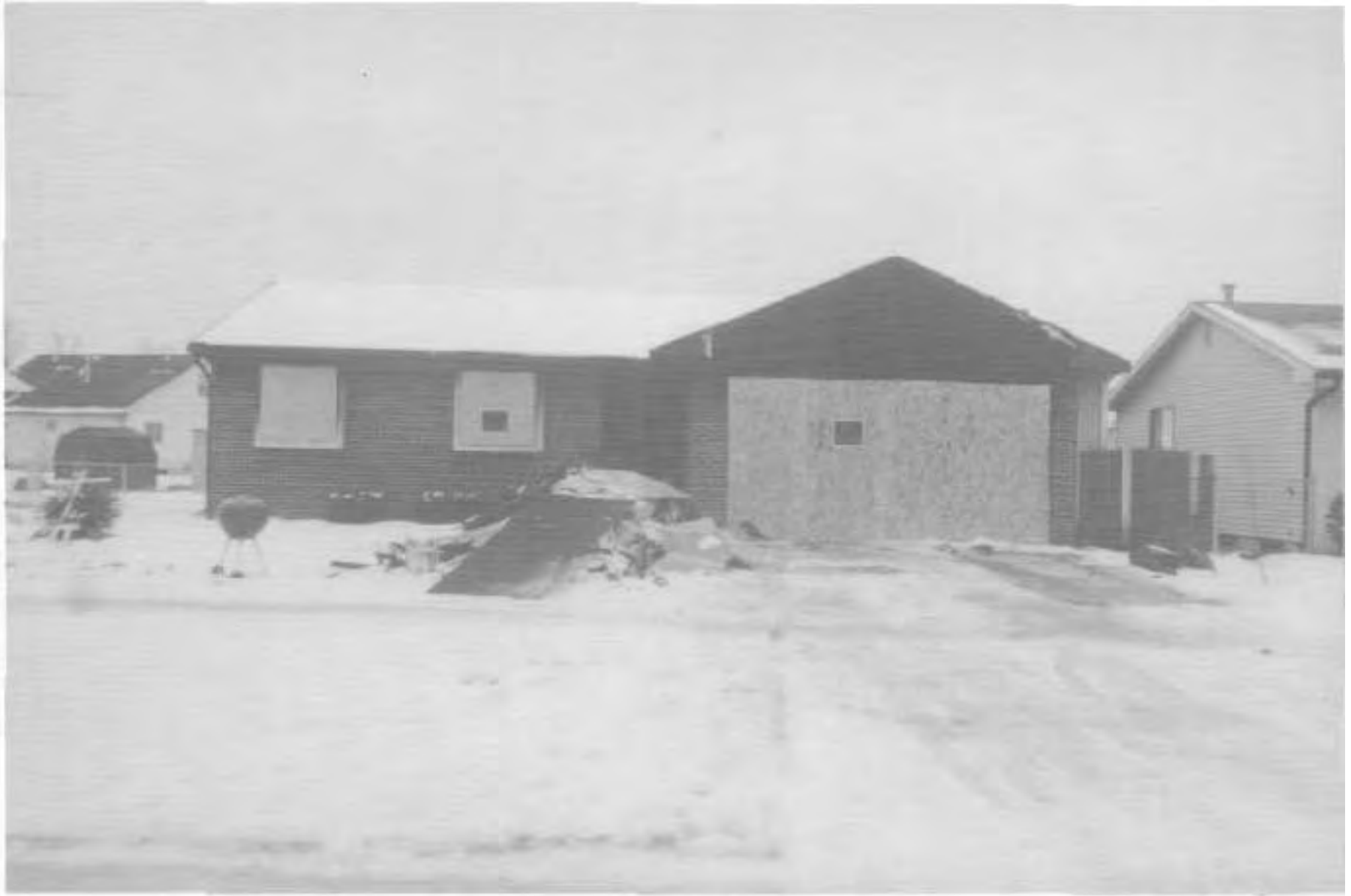
Front view of the Dell'Orco home, with evidence of fire venting through the garage door opening.
