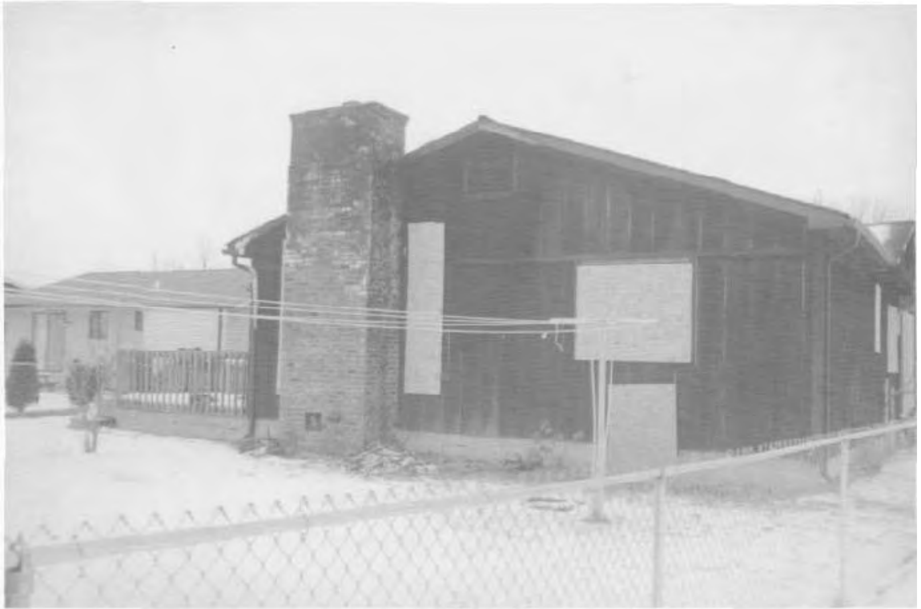
Rear view of the home, with no evidence of fire venting through the rear bedroom window.
