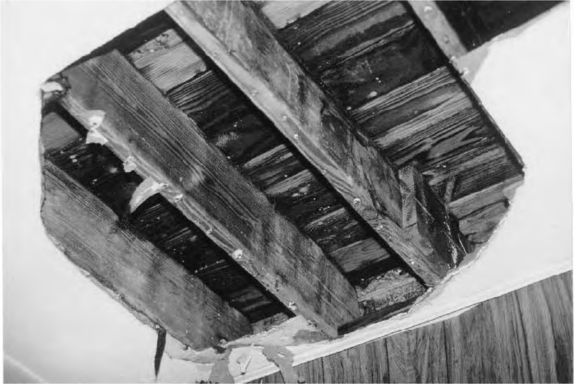
Typical floor construction, shown from ceiling of first floor room.
