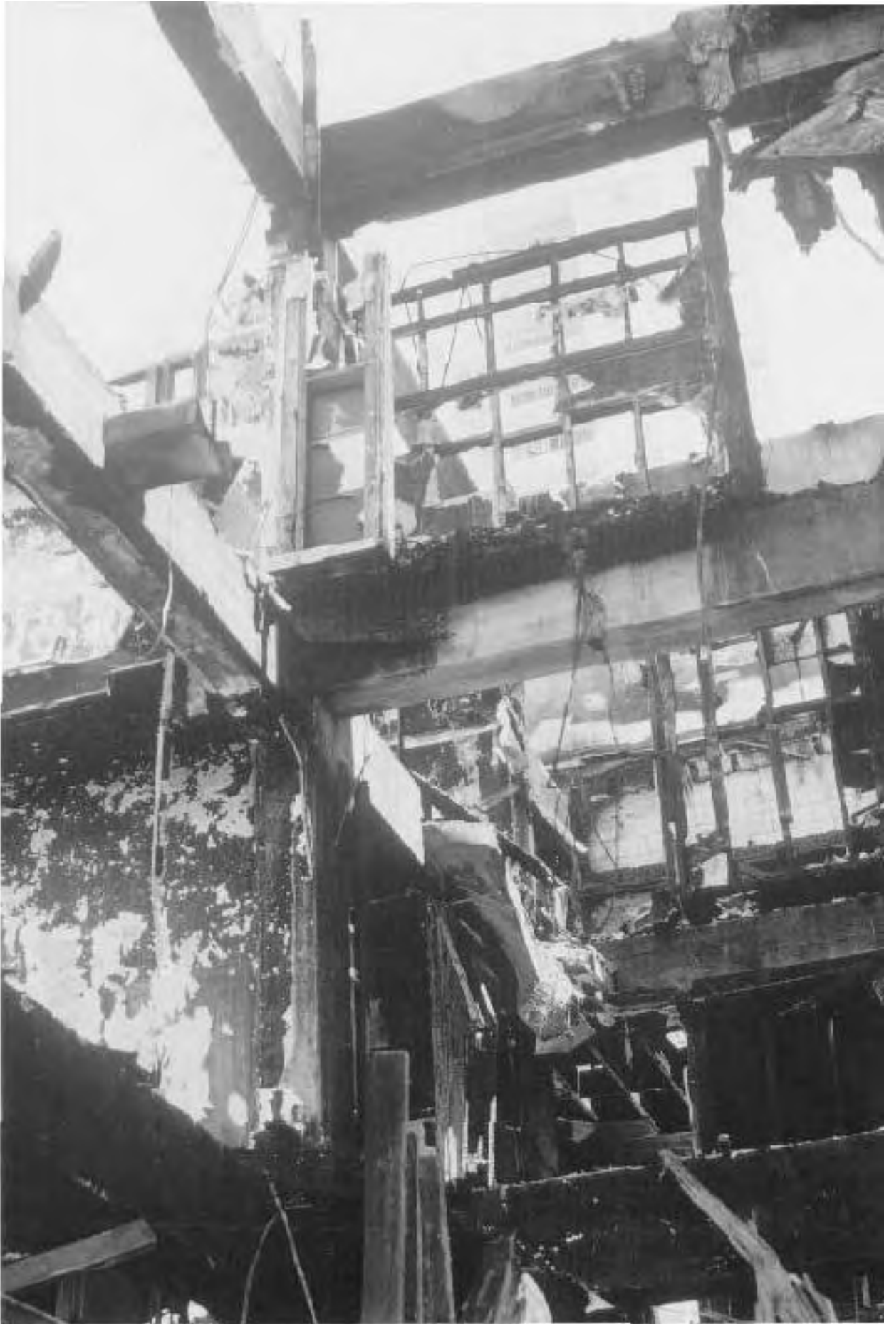
Lobby, looking up through roof facing Collins Street.
