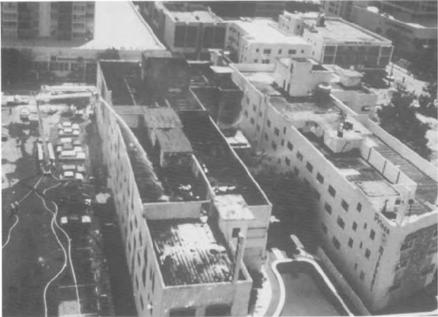
Aerial view of Hotel after the fire. Note destruction of the roof and proximity of the Prince Michael Hotel. (MBFD photo)
