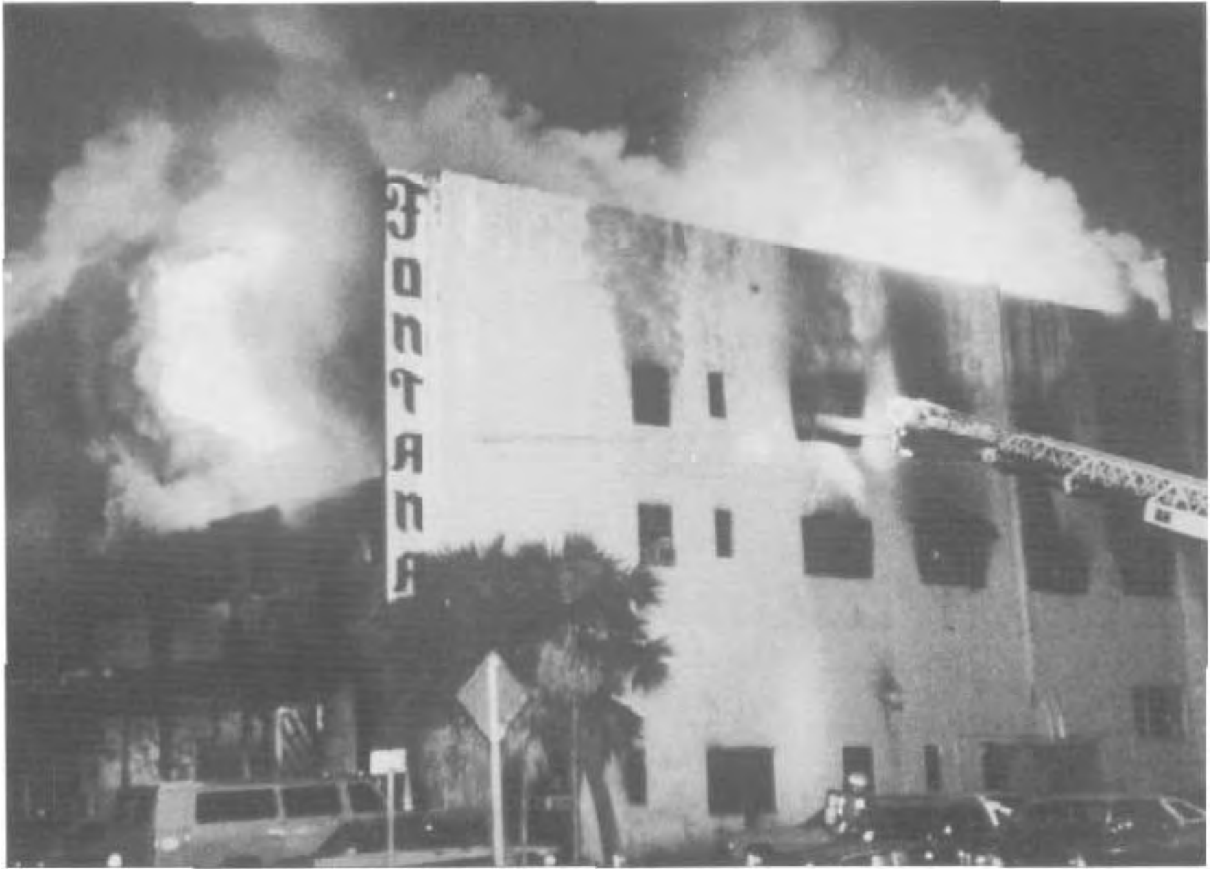
Exterior attack in progress, note fire involvement of attic.
