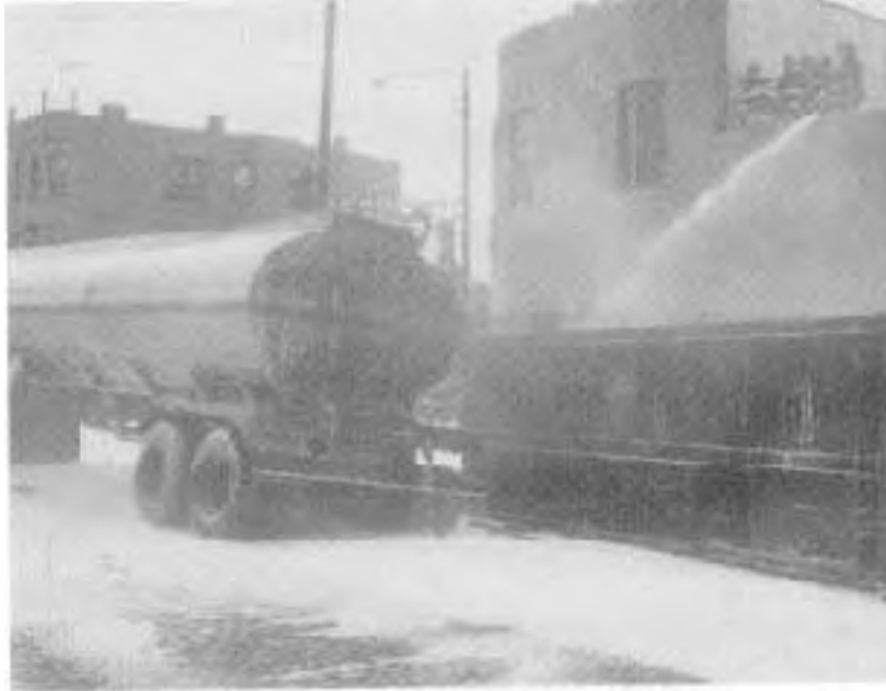
11. Firefighters flood debris in dumpster to prevent reignition of gasoline.
