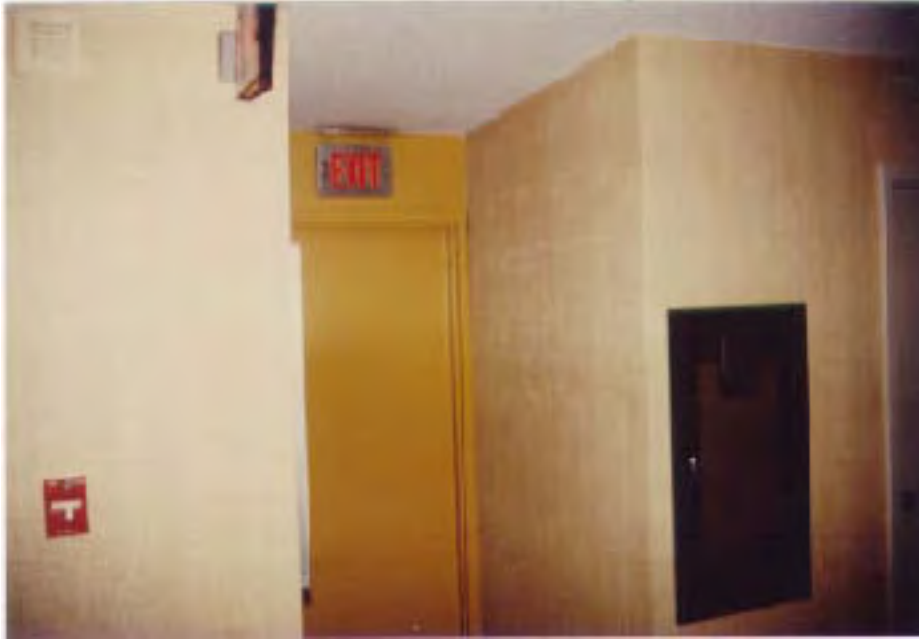
Figure 6. Entrance to exit Stairway 2 -- 9th floor. Compare with Figure 7 after fire.
