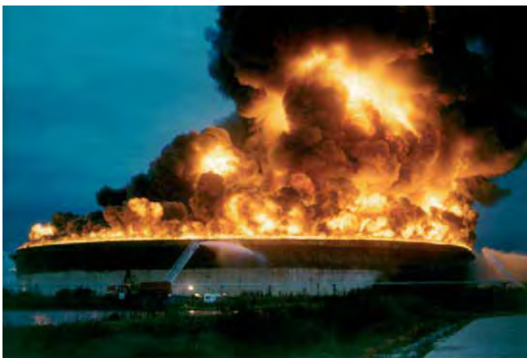
The Orion Tank Fire in 2001, world record in tank fire fighting. Photo courtesy of Industrial Fire World
