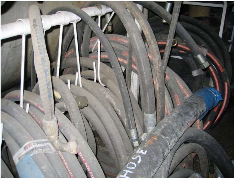
Figure A 9 Photos taken during the visit to the Hallandsåstunnel.
