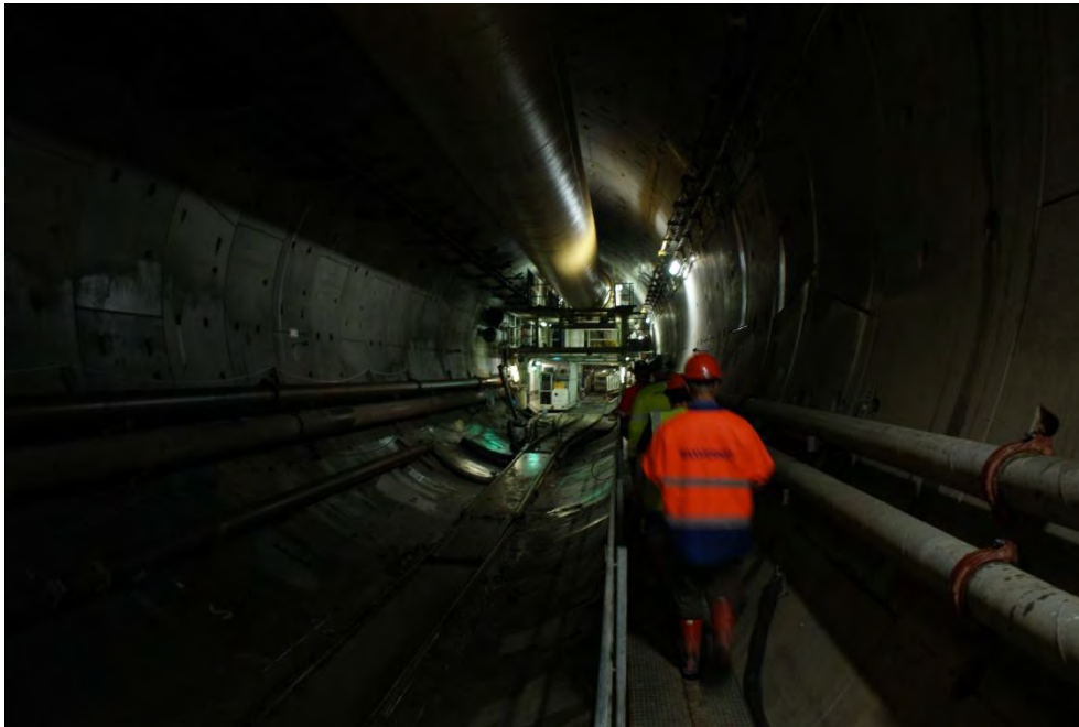
Figure A 6 The rear end of the TBM machine in the Hallandsås tunnel.
