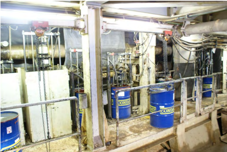
Figure A 8 Photos taken during the visit to the Hallandsåstunnel.
