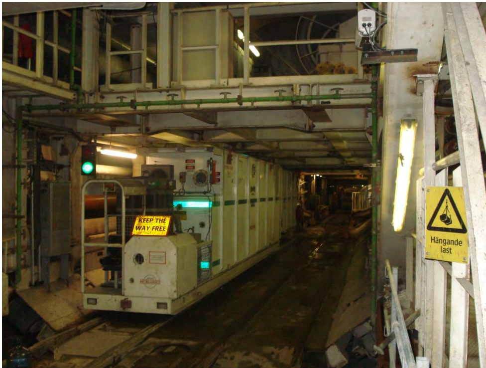
Figure A 7 The rescue train on the TBM drilling machine.
