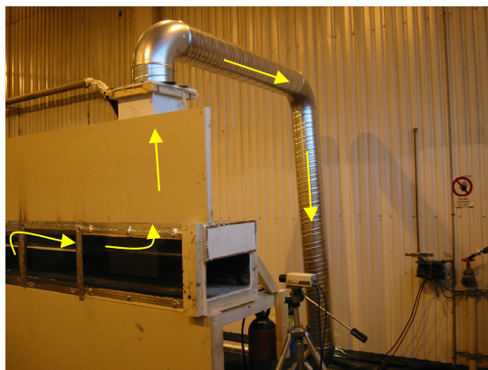
Figure 3 A photo and a schematic drawing of the exhaust ventilation used in the tests to measure the HRR.
